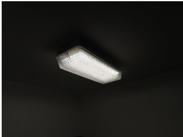
Photo showing the LED panel type emergency light Wang Chi House (Photo taken on 1.12.2025)
