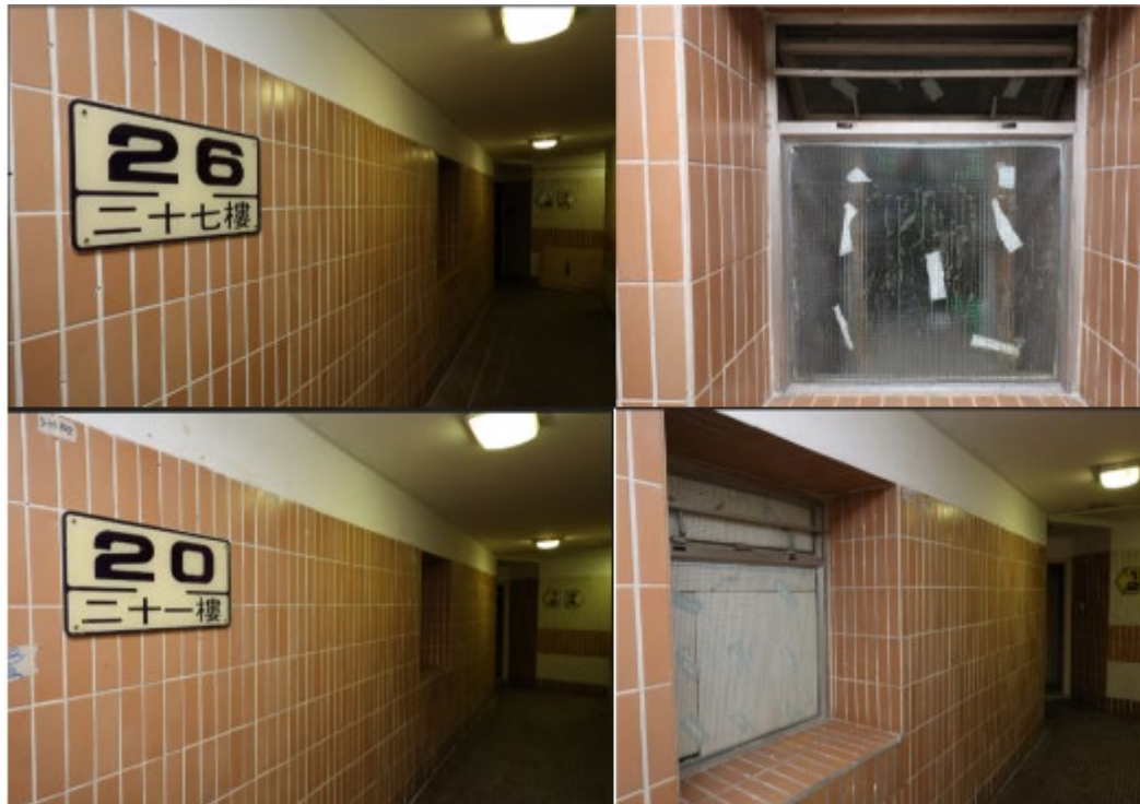
Photo: One large, fixed window and aThe upper part of the windows at the lift lobbies is smaller and openable, while the lower part of the windows is larger and fixed. The majority of the windows at the lift lobbies of different floors are typically left open, promoting ventilation across residential areas. Some of such windows were covered with foam boards.
