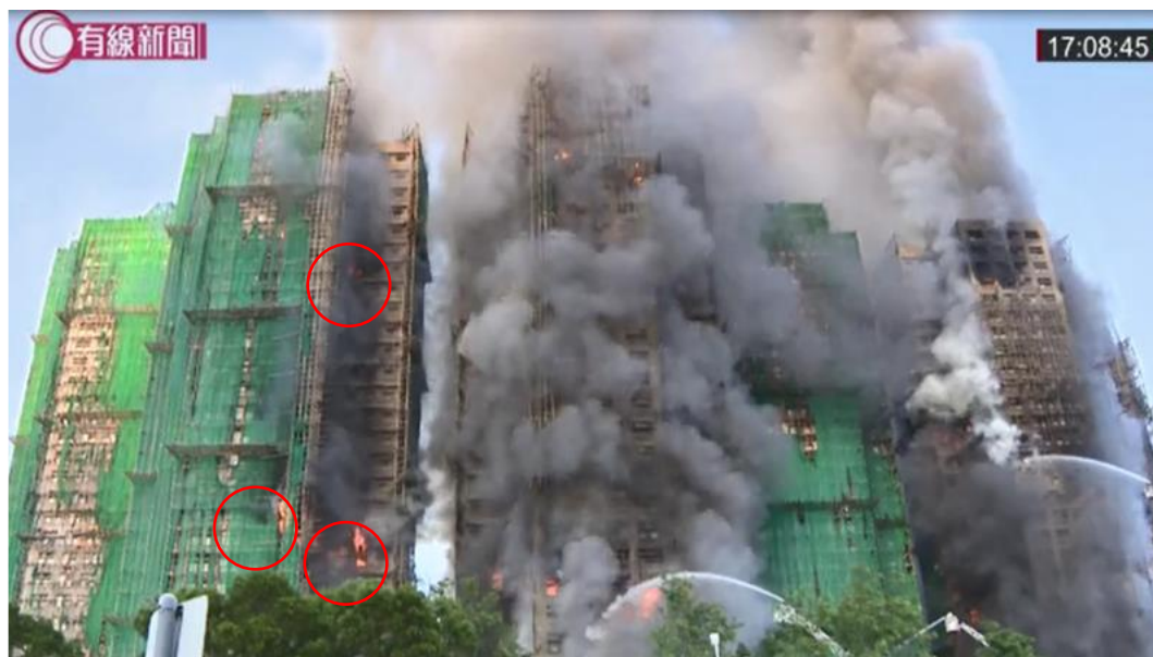
Photo 8-4 (b): Visible Flames in Flats 1202, 1203 and 2202 of Wang Tao House 112
