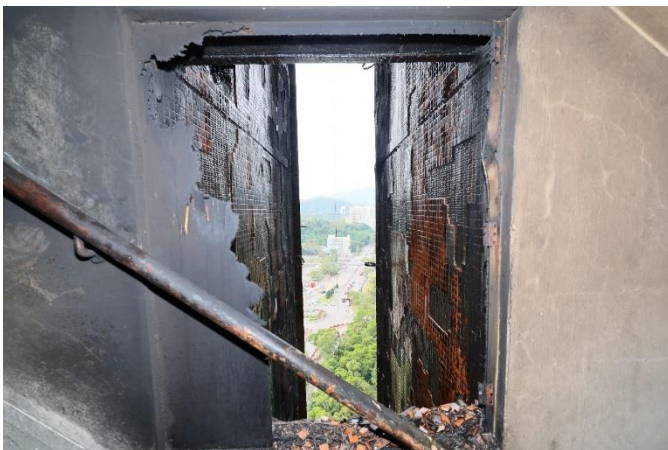
Wang Tai House Rear staircase between 25/F & 26/F
