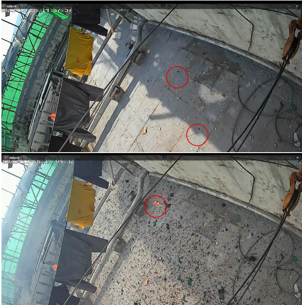
Photos 8-16 (a) & (b): Embers Falling From a High Level Observed on the Roof of Wang Tai House
