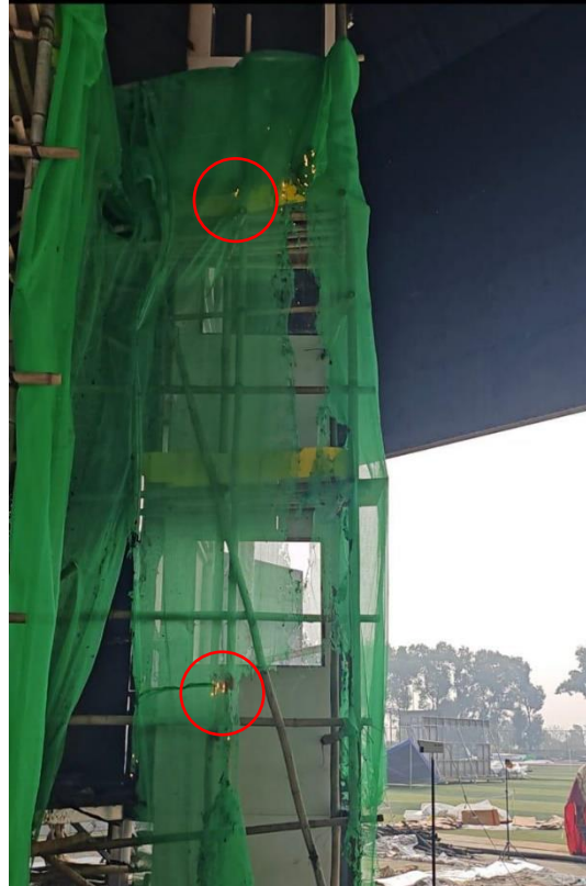
Photo 7-5 (b): Flaming Droplets Dripping and Spreading Fire
