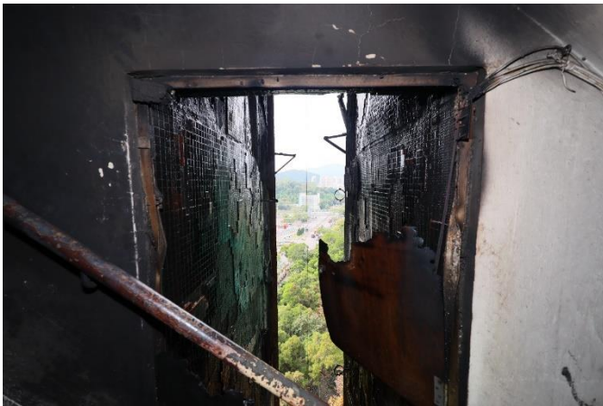
Wang Tai House Rear staircase between 15/F & 16/F
