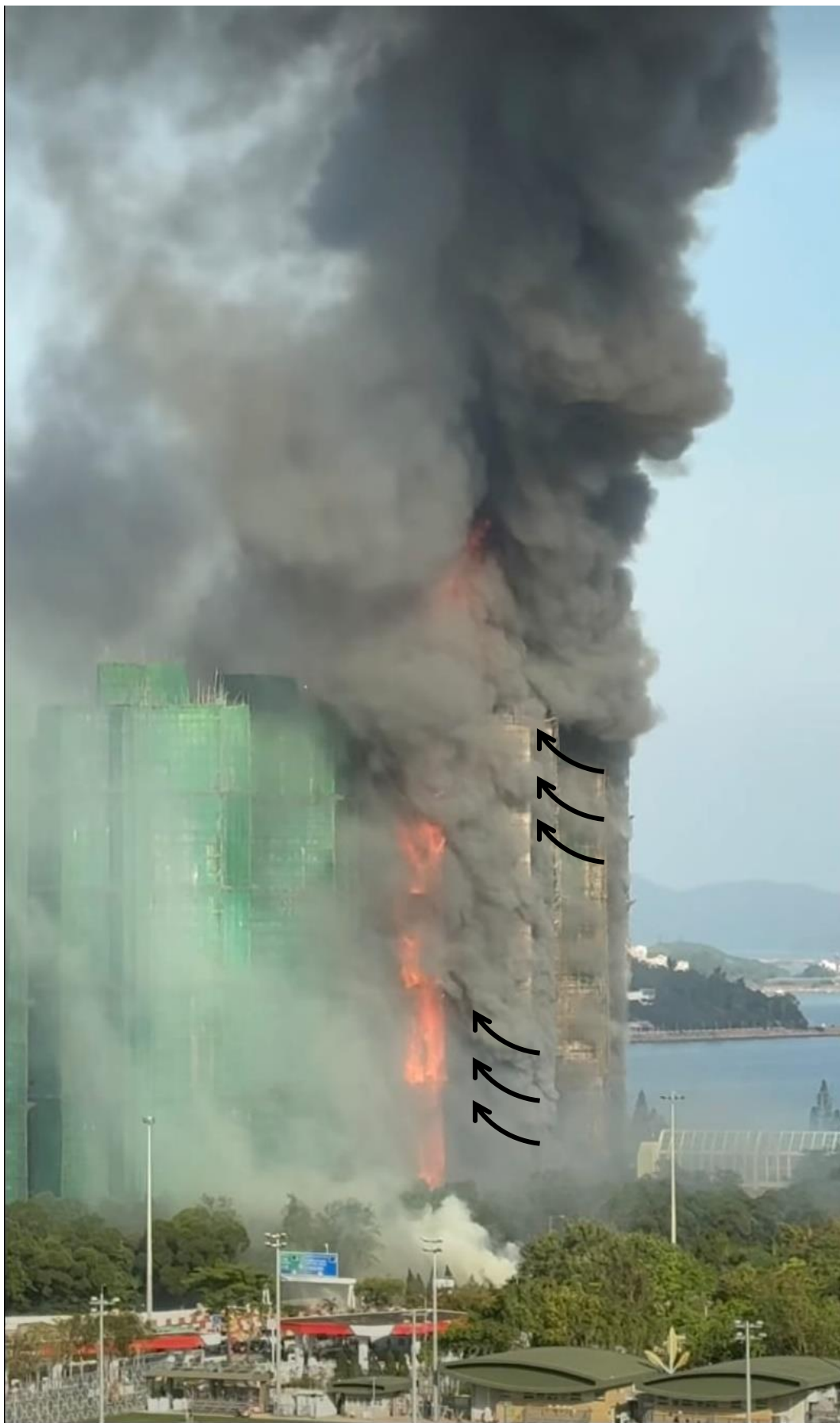
Photo 7-10 (c): Heavy Smoke From Wang Cheong House & Wang Tai House
