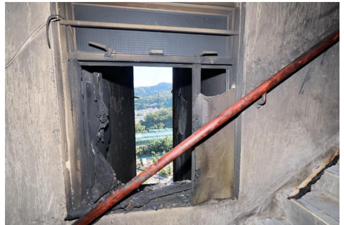
Wang Sun House Rear staircase between 19/F & 20/F
