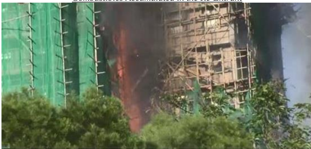
Photo 6-7 (d): Flaming Fire Observed in the Lower Portion of Wang Tao House
