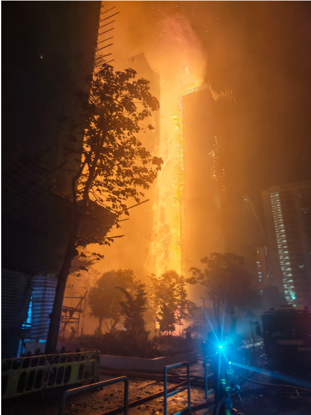
Photo 8-9: Rapid Fire Spread Observed at the Re-Entrant Between Flats 02 and 03 of Wang Yan House
