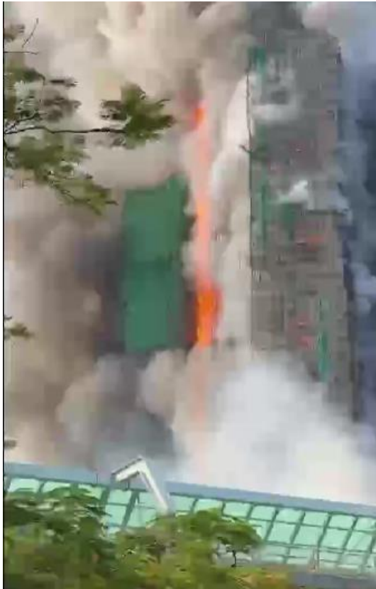
Photo 5-10 (a): Fire Spread Along the East Re-Entrant of Wang Tai House at 1516 Hours
