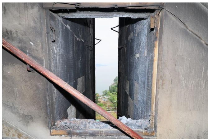
Wang Cheong House Front staircase between 20/F & 21/F
