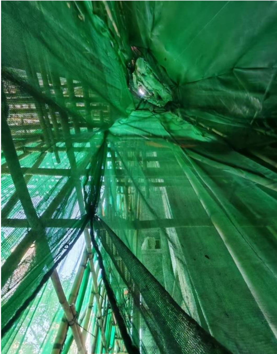
Photo 4-13: Triangular Channel Leading From the Flat Roof to R/F at the Re-Entrant
