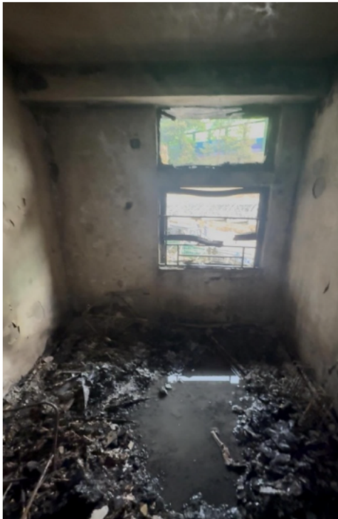
Bedroom 1 of Flat 105 Overview (Photo B11)
