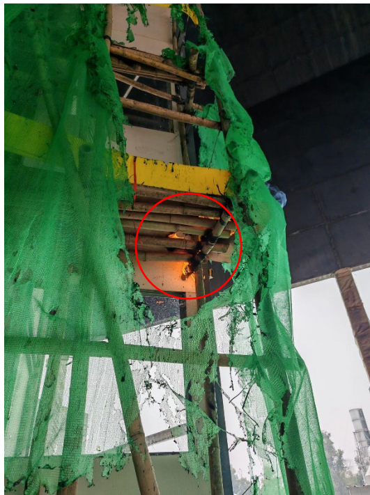
Photos 2-17 (g) & (h): Flaming Droplets Causing Further Fire Propagation.
