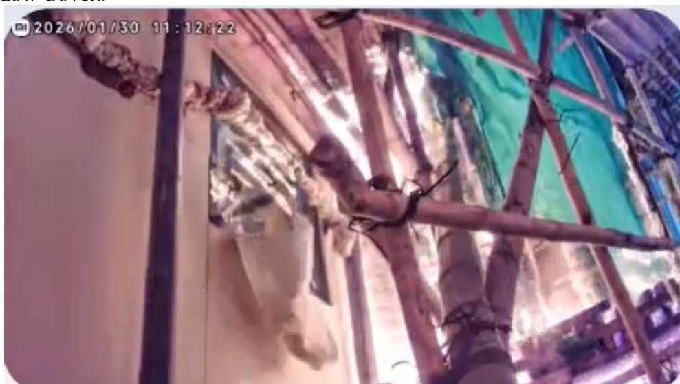
Photo 2-13 (c): Fallen Polystyrene Window Covers Potentially Sparking Secondary Fires
