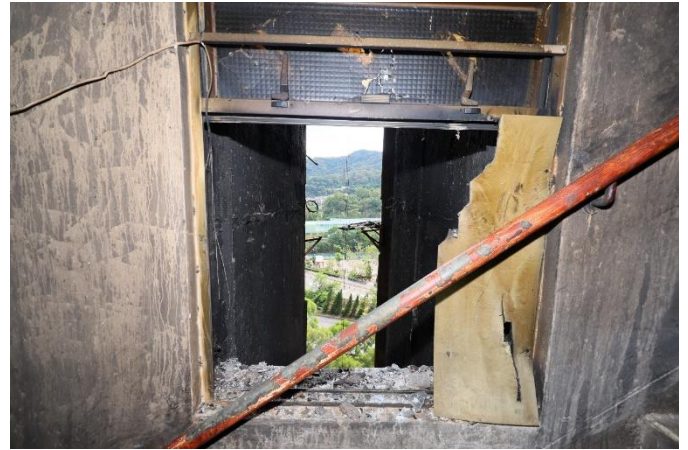
Wang Sun House Front staircase between 10/F & 11/F
