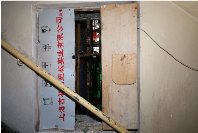
Wang Yan House Rear staircase between 3/F & 4/F
