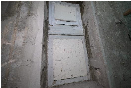
Photos 4-14 (a) to (c): Polystyrene Window Covers
