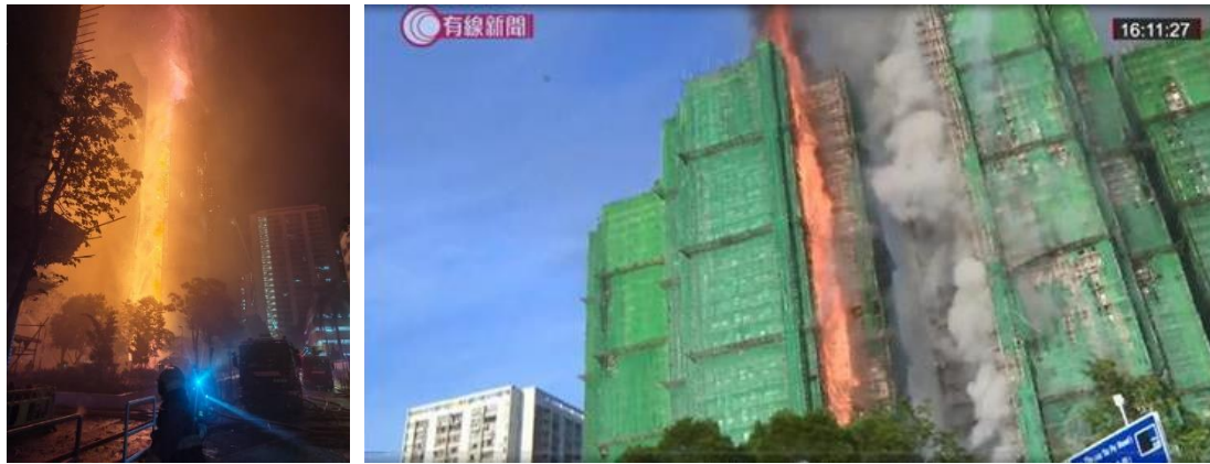
Photos 8-1 (a) & (b): Rapid Vertical Fire Spread Along the Re-Entrant Observed in Wang Tao House and Wang Yan House
