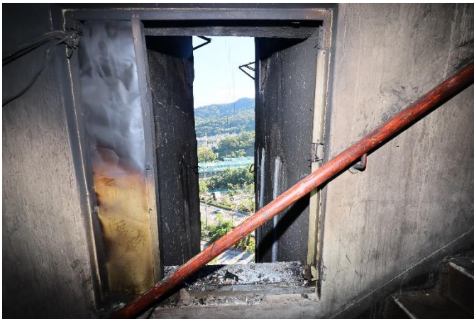
Wang Sun House Rear staircase between 15/F & 16/F
