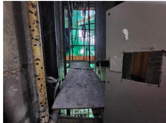
Photo 4-8: Toe-Boards on the Working Platforms Inside Scaffolding
