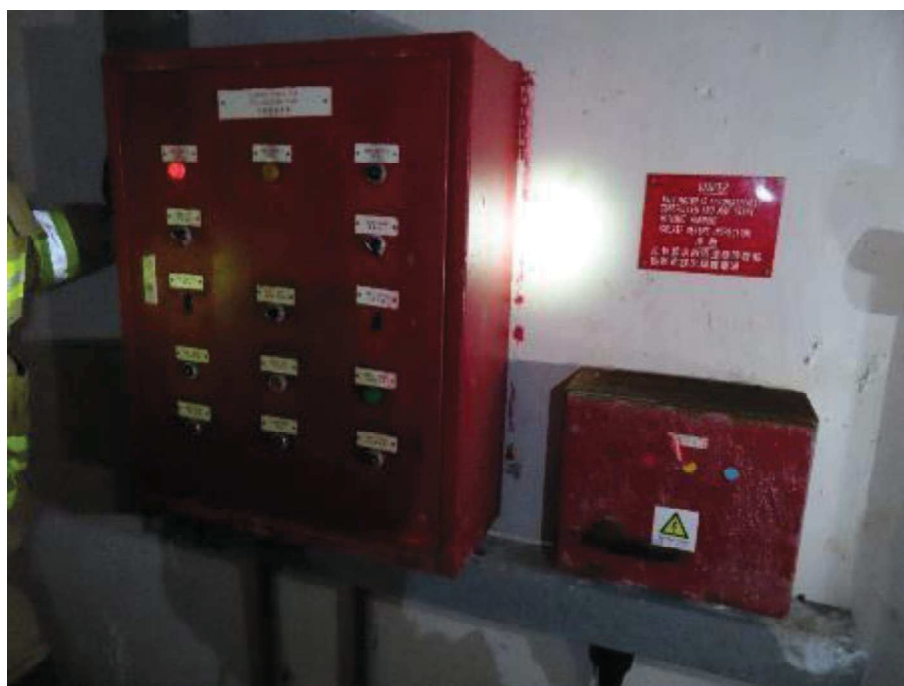
Photo showing the control panel of fire booster pump (Power available after switch on)
