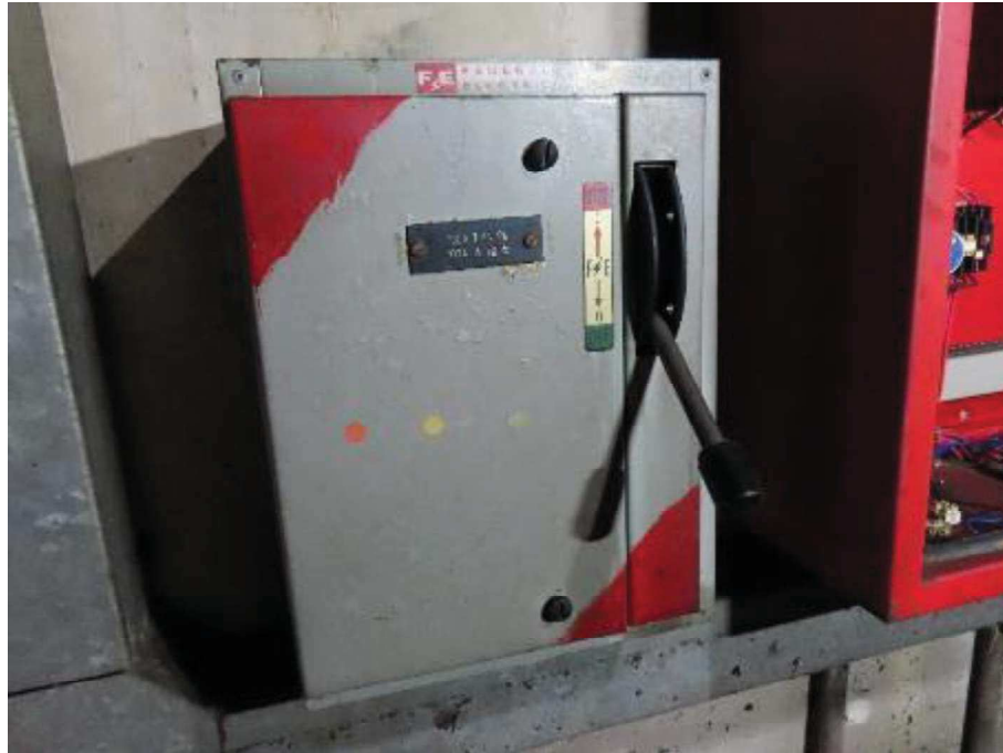
Photo showing the 100A TPN switch of fire booster pump panel (Power off position)
