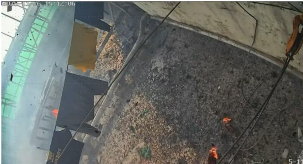
Photos 6-9 (a) & (b): Flying Embers Suspected Spreading From Wang Cheong House to Wang Tai House at About 1506 and 1511 Hours 73
