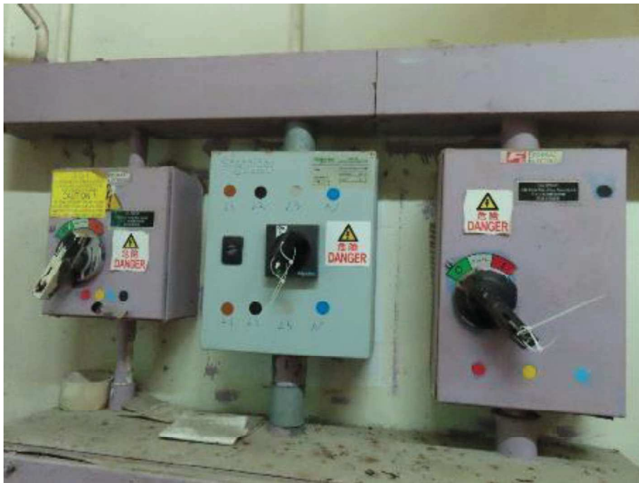
Photo showing the main switch of upfeed water pump (Power on position)
