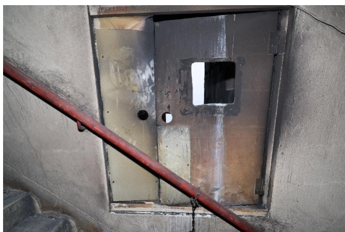
Wang Cheong House Rear staircase between 25/F & 26/F
