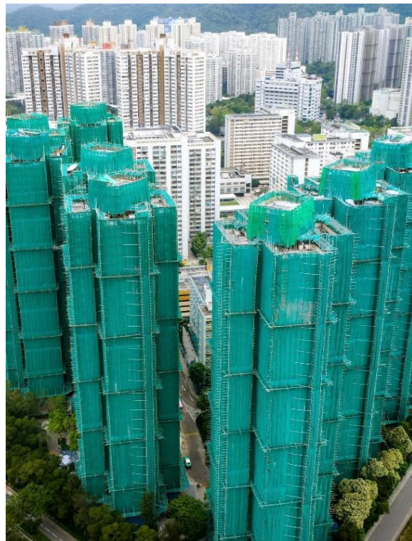
Photos 6-11 (a) & (b): Buildings in Wang Fuk Court Enveloped by Safety Nets
