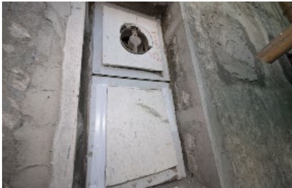
Photo: Bathroom windows of Unit 102 were covered externally by foam board
