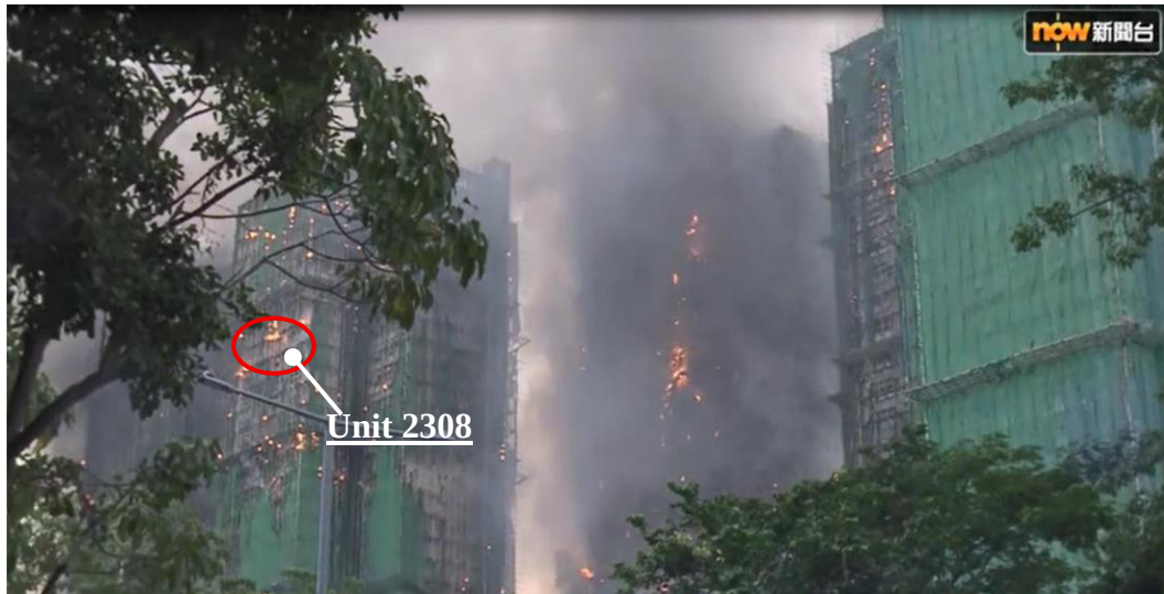
Photo 8-7 (c): Combustible Building Envelope Outside Flat 2308 of Wang Kin House on Fire at 1605 Hours
