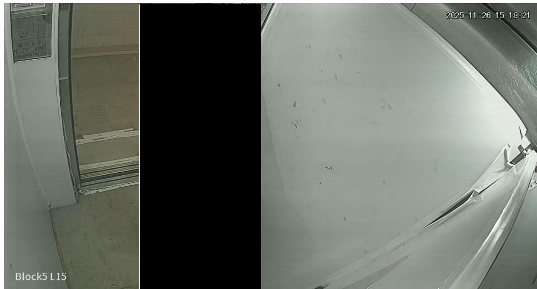
Photo 10-4 (b): CCTV Footage of Lift L15 on the G/F at 1520 Hours
