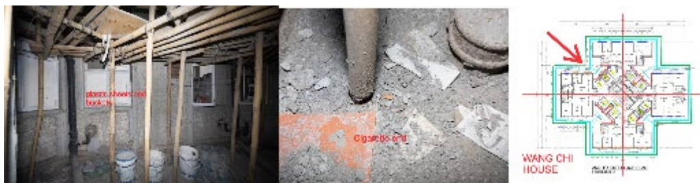
Photo: Re-entrant between Units 102, 103 and meter room
