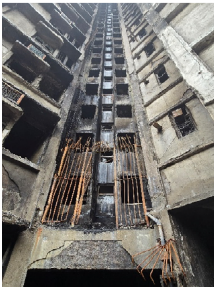
Lightwell Platform (Photo R1)
