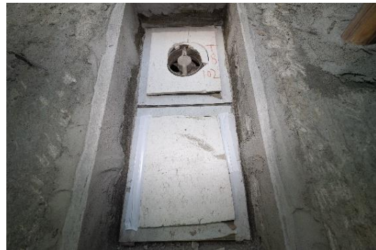
Photos 4-14 (a) to (c): Polystyrene Window Covers
