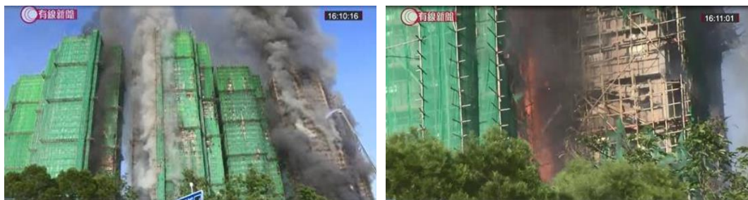
Photos 8-18 (b) & (c): Flaming Fire Observed in the Lower Portion of Wang Tao House at 1611 Hours
