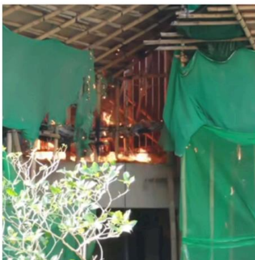
Fig. 2.11 Picture of initial fire incident
