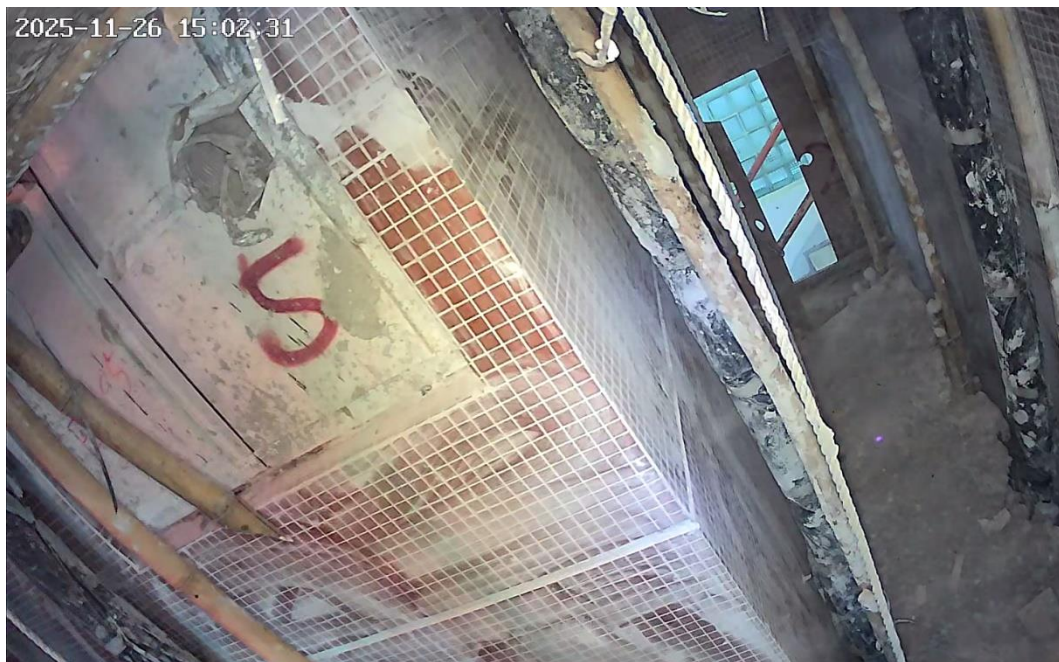
Photo 5-9 (b): A Reflection of the Fire was Captured by CCTV Installed on the Scaffolding of Wang Tai House at About 1503 Hours 46
