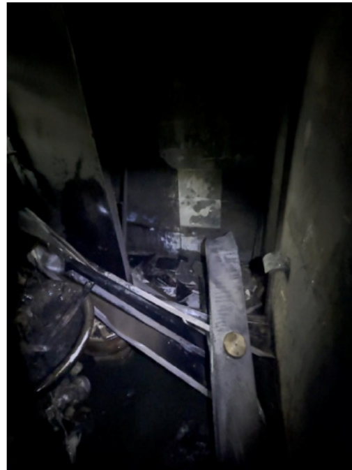
Bathroom of Flat 104 Overview (Photo A12)
