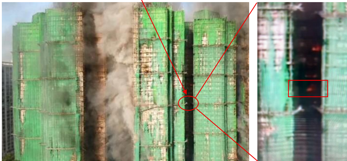
Photo 8-8 (a): External View of Flat 02, Wang Kin House at 1619 Hours
