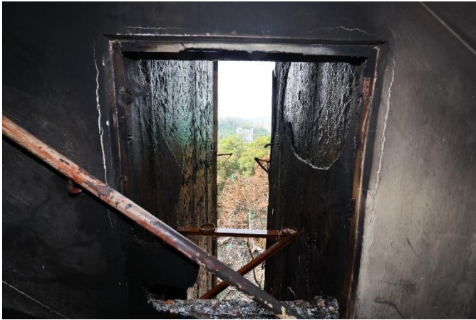
Wang Tai House Rear staircase between 5/F & 6/F
