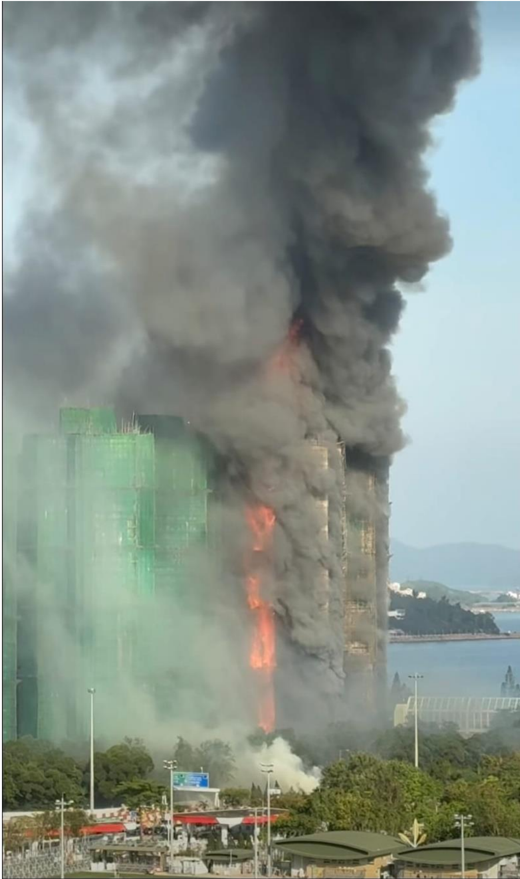
Photo 5-11: Rapid Fire Spread at the West Re-Entrant of Wang Tai House
