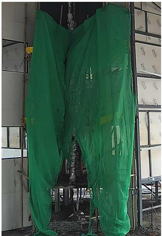
Photo 2-12 (c): Post-Fire Condition in Test 4 using FR Safety Nets
