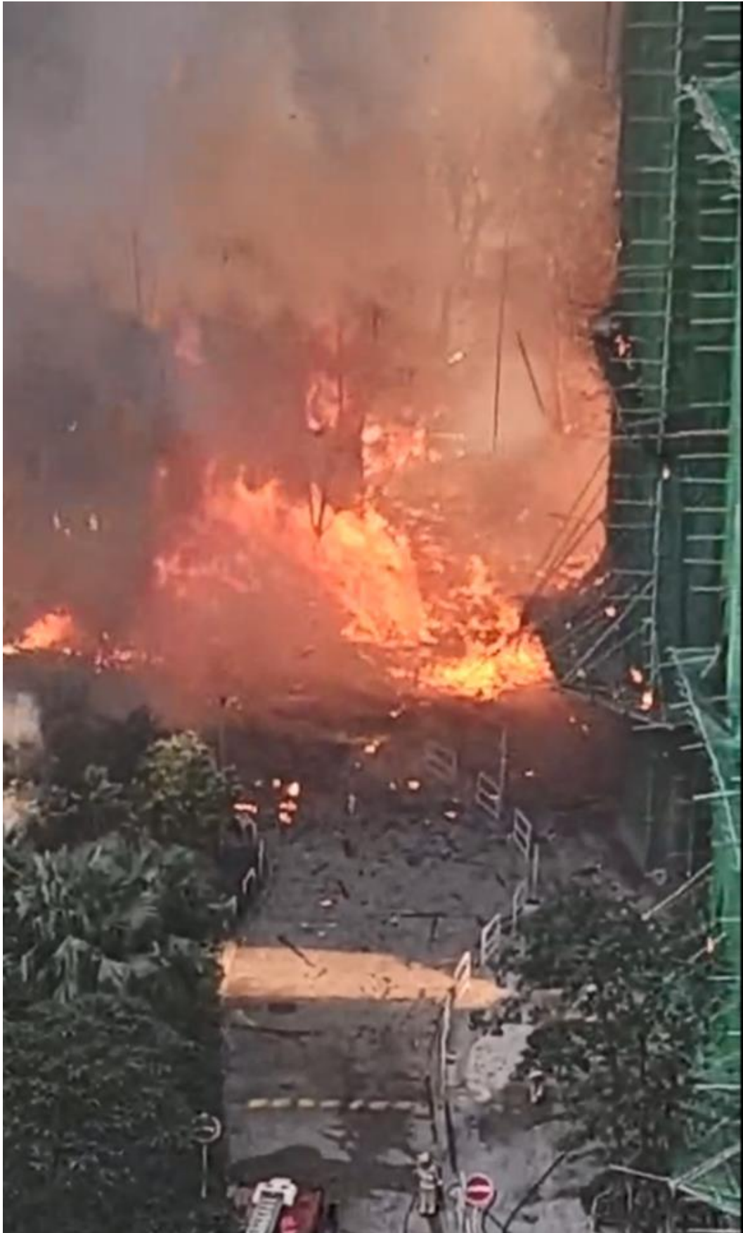
Photo 10-3 (b): Flaming Bamboo Scaffolding and Other Construction Materials Detached From the Upper Levels
