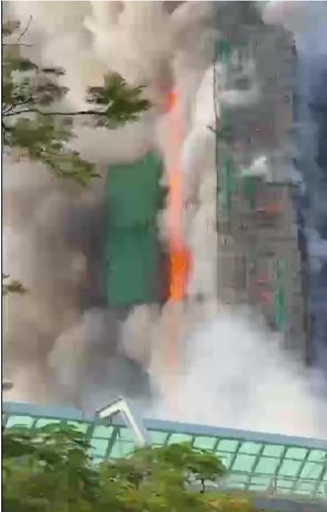
Photo 10-7 (e): Rapid Fire Spread at the East Re-Entrant of Wang Tai House at 1516 Hours
