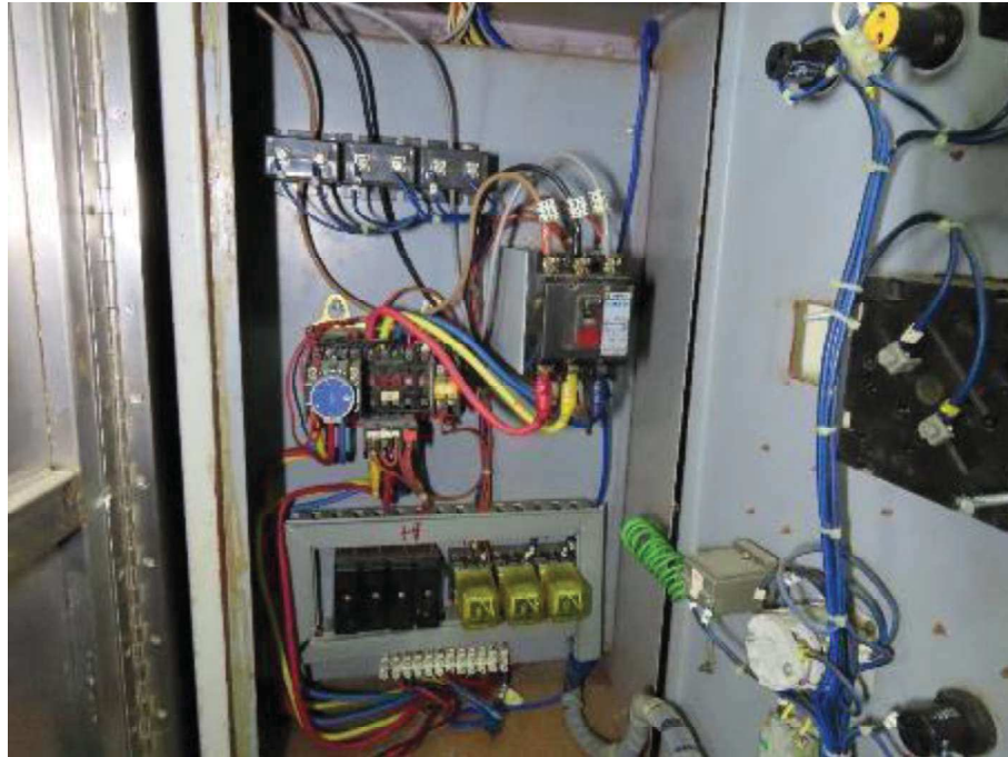
Photo showing the power breaker of the control panel of upfeed water pump (Power on position)
