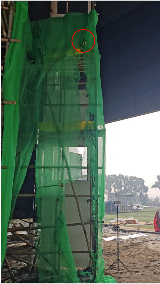
Photo 2-17 (a): Small Fires Spreading Along Safety Nets, Forming Flaming Droplets
