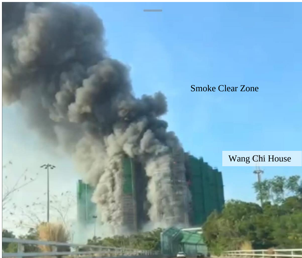
Photo 7-11: Smoke Clear Zone Above Wang Chi House
