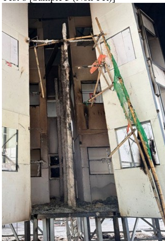
Photo 2-16 (l): Post-Fire Condition in Test 9 [Sample 4 (Wang Chi House)] [35]
