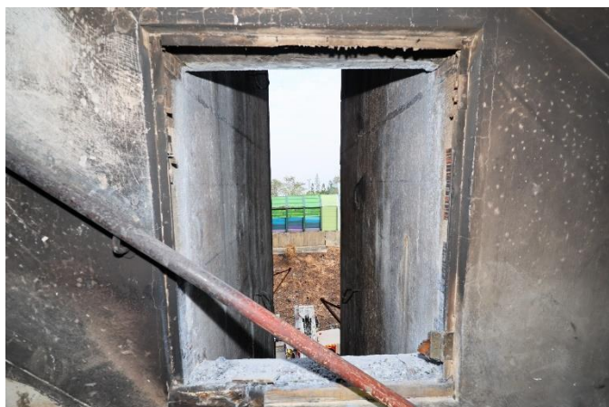
Wang Cheong House Rear staircase between 5/F & 6/F
