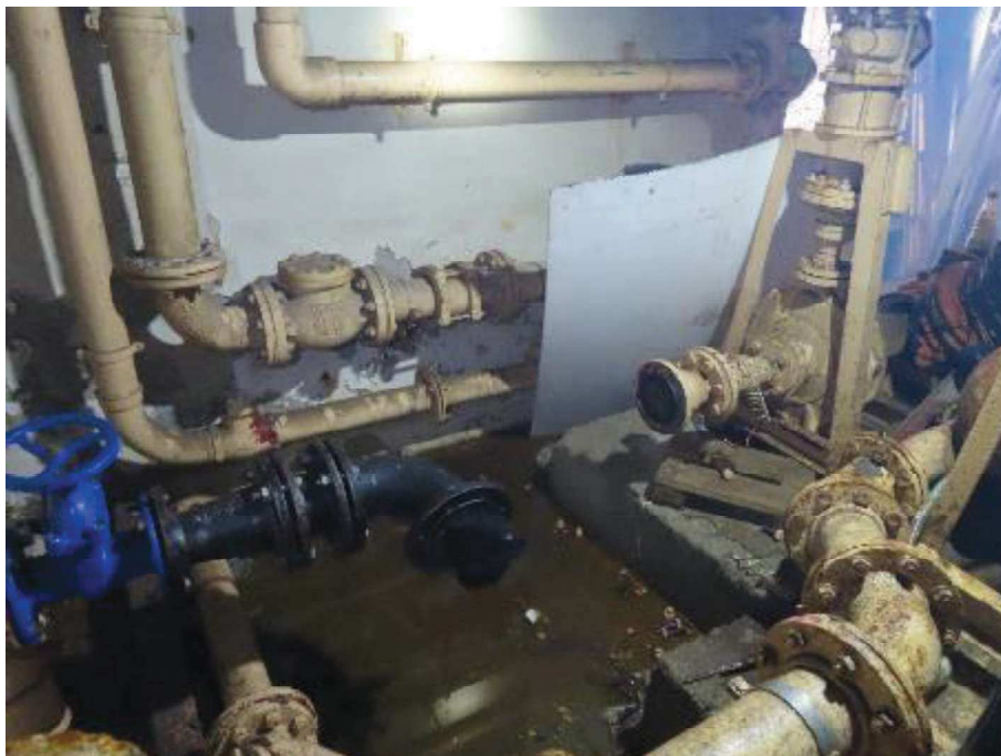
Photo showing the upfeed water pump
