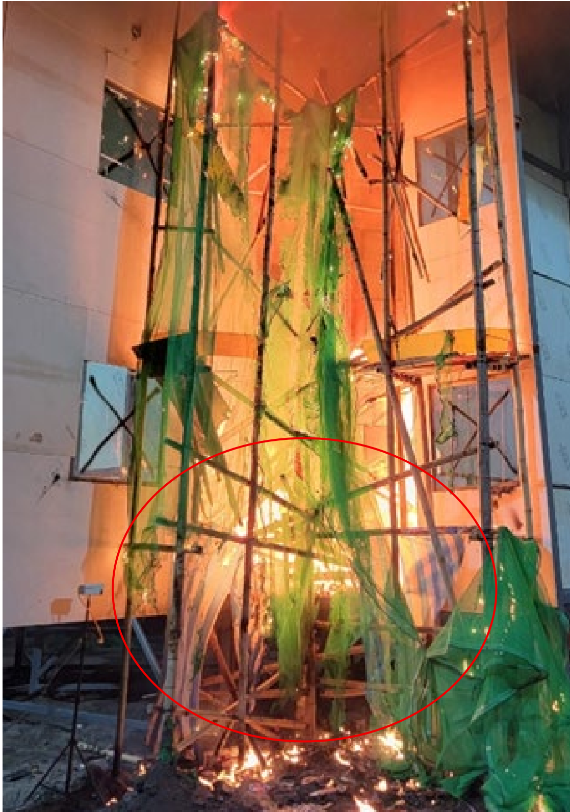
Photo 4-6: Collapsed Burning Bamboo from the Damaged Bamboo Scaffolding in Fire Test
