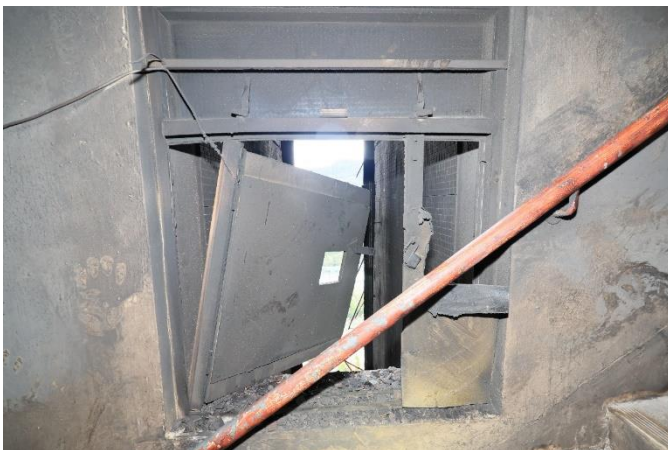
Wang Sun House Front staircase between 24/F & 25/F
