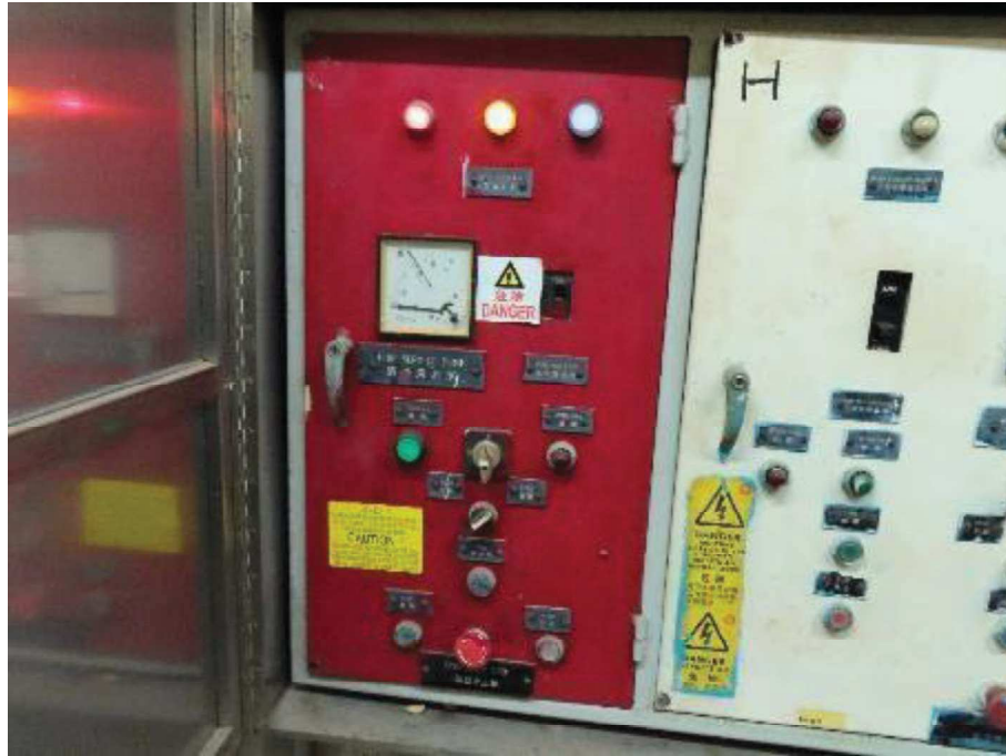
Photo showing the control panel of upfeed water pump (Power unavailable)
