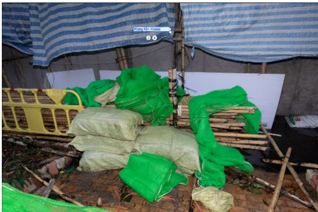
Photo: Safety net and bamboo outside Wang Kin House
