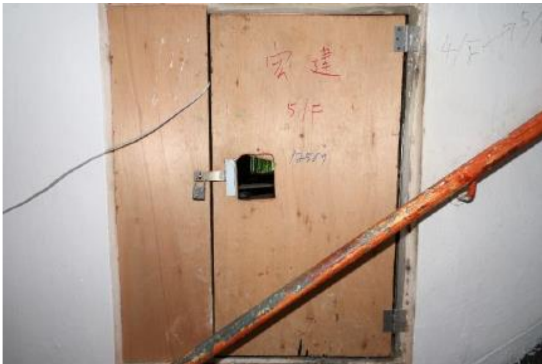
Photos 4-9 (a) to (c): Replacement of Windows With Movable Board
