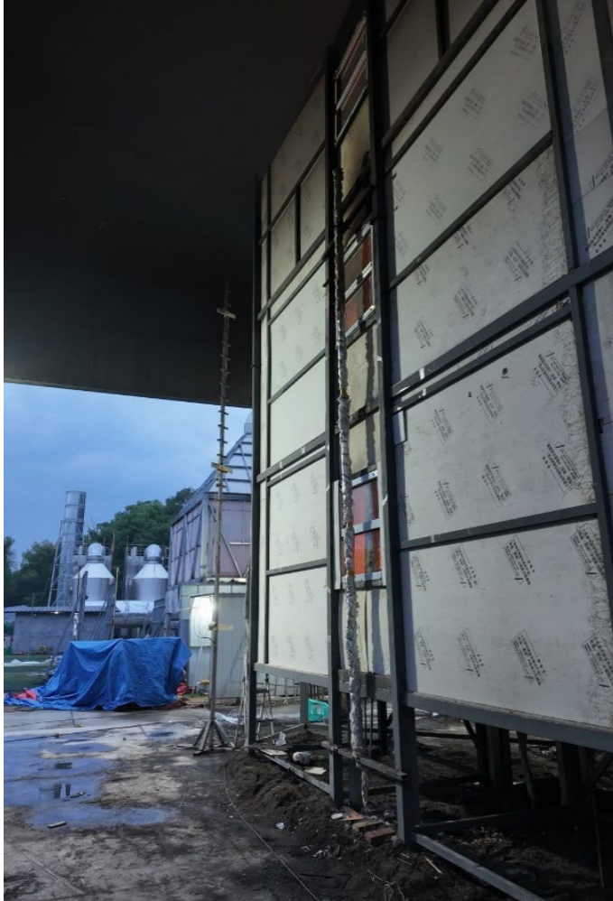
Photo 2-18 (h): Condition of Fire-rated Glass during Test 13
