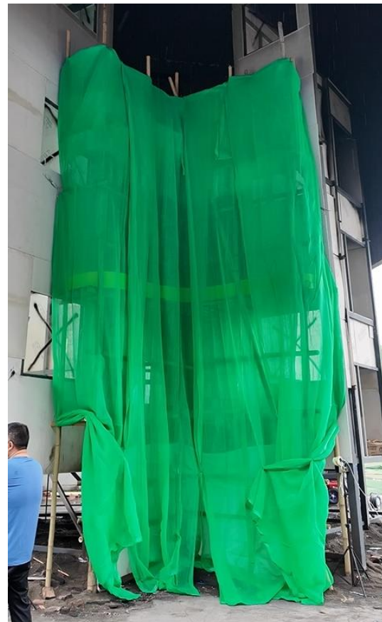
Photo 7-6 (b): Post-Fire Condition in Test 11 Using FR Safety Nets and FR Canvas
