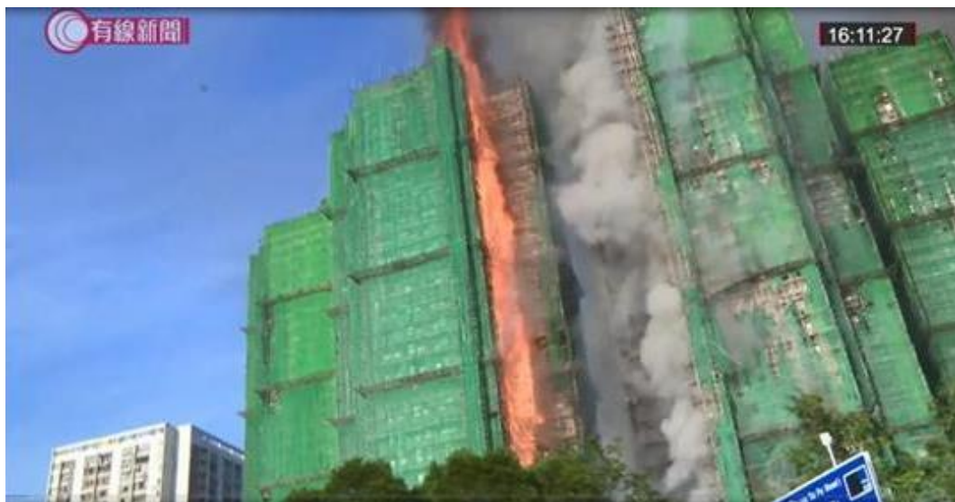
Photo 8-18(d): Fire Spread Vertically Throughout the Re-Entrant of Wang Tao House
