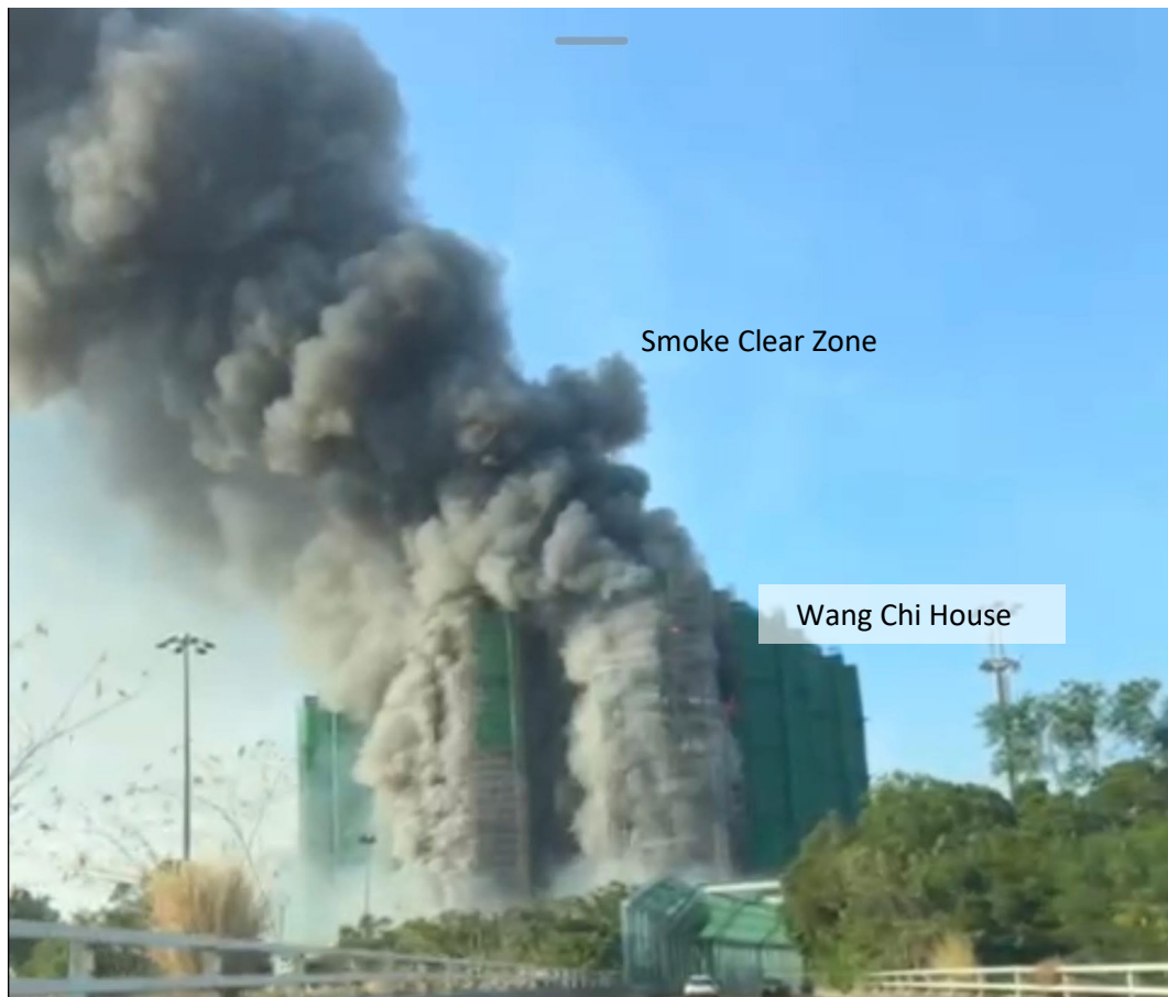
Photo 3-2: Smoke Clear Zone Above Wang Chi House
