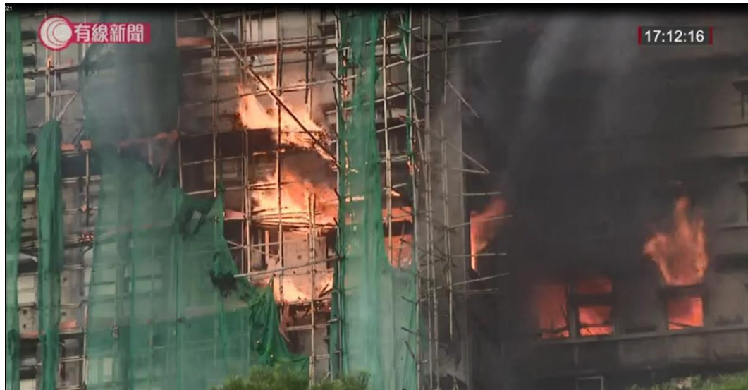
Photo 10-6 (a): Polystyrene Panels Fueling Fire Spread on the Building Façade
