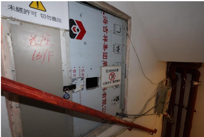
Wang Chi House Front staircase between 14/F & 15/F
