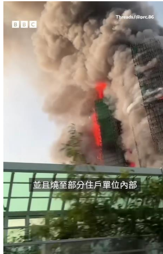
Photo 5-10 (b): Fire Spread Along the South Re-Entrant of Wang Tai House at 1517 Hours
