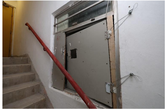
Wang Chi House Rear staircase between 9/F & 10/F
