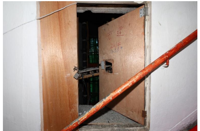
Wang Kin House Rear staircase between 19/F & 20/F
