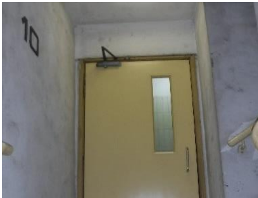
Photo 4-1 (c): Staircase Landing of 10/F, Wang Kin House (Before the Renovation Works)
