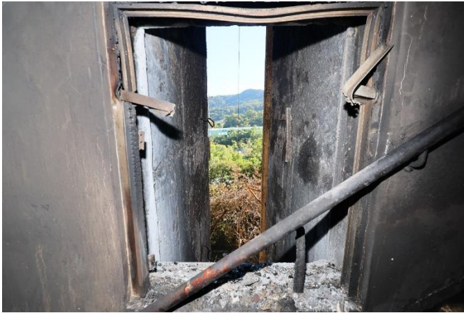
Wang Sun House Rear staircase between 5/F & 6/F
