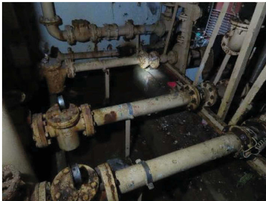
Photo showing the piping of upfeed water pump (Connected)
