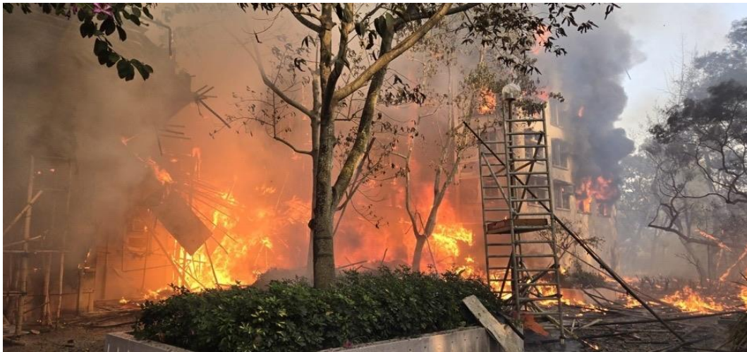
Photo 10-3 (a): The Burning Debris and Bamboo Scaffolding Blocking Exits
