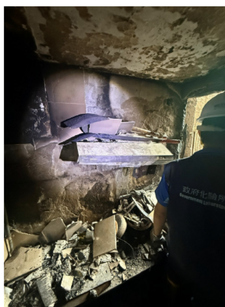
Range Hood in Kitchen of Flat 105 (Photo B2)
