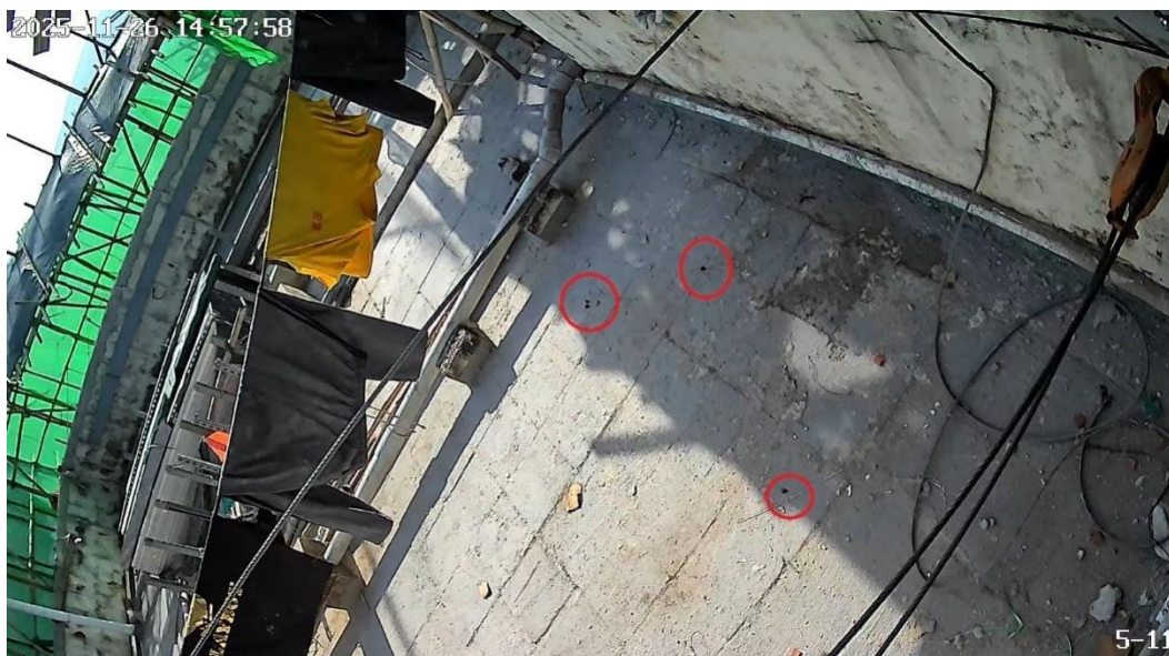
Photo 5-9 (a): Flying Embers Observed on the R/F of Wang Tai House at About 1458 Hours 45
