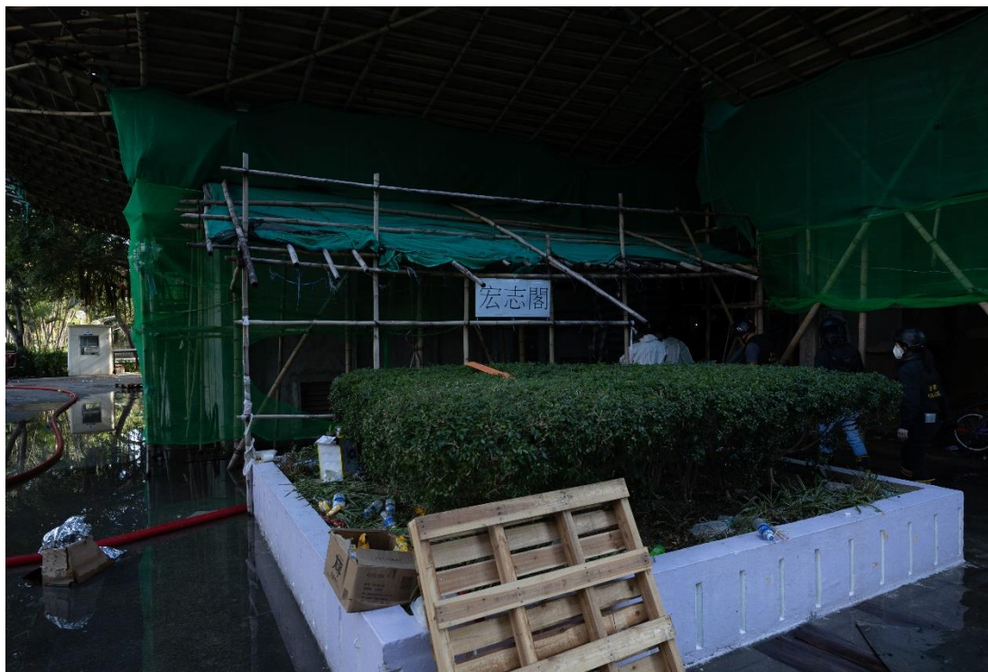
Photo 4-11 (c): Printed Building Signage at Wang Chi House
