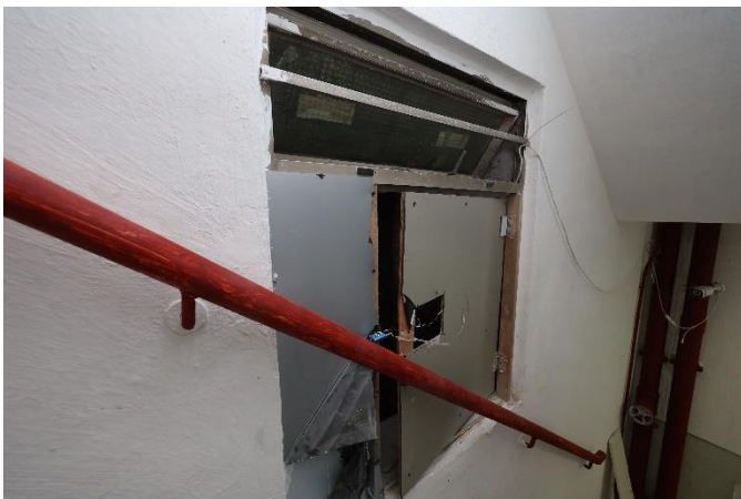
Wang Chi House Front staircase between 24/F & 25/F
