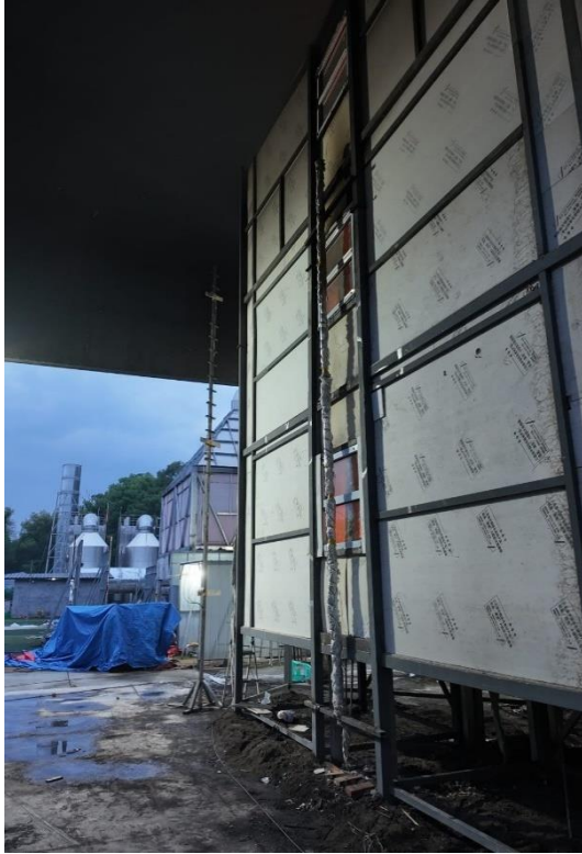
Photo 7-9: Condition of Fire-rated Glass During Test 13
