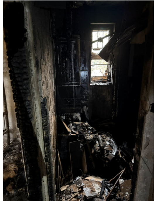
Bathroom of Flat 105 Overview (Photo B14)
