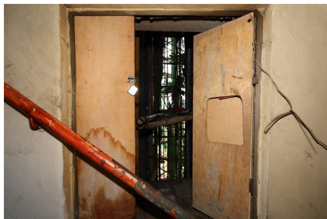
Wang Tao House Front staircase between 20/F & 21/F
