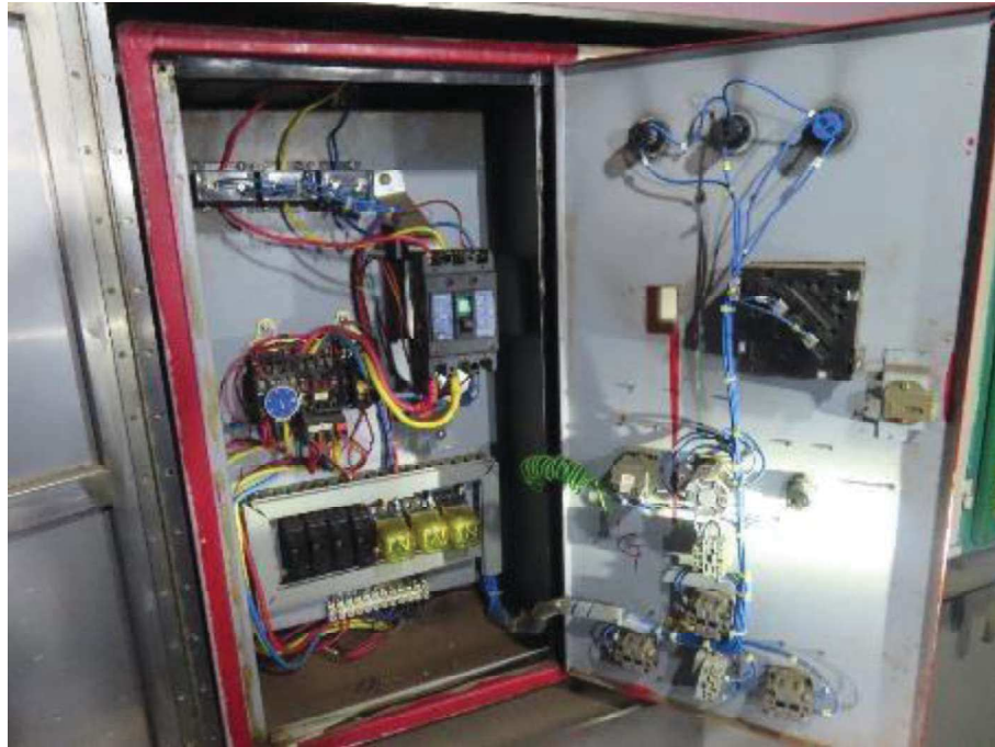
Photo showing the power breaker of the control panel of upfeed water pump (Power off position)
