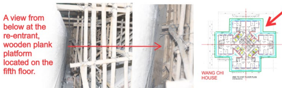
Photo: A view from below at the re-entrant between Units 104, 105 and staircases
