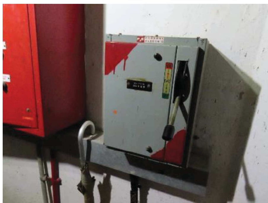
Photo showing the 100A TPN switch of fire booster pump panel (Power off position)
