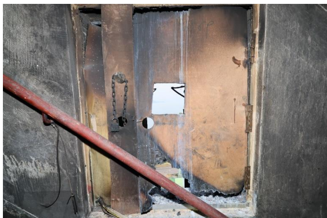
Wang Cheong House Rear staircase between 15/F & 16/F
