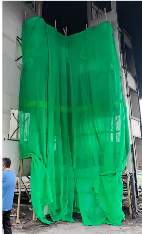
Photo 2-18 (b): Post-Fire Condition in Test 11 using FR Safety Nets and FR Canvas
