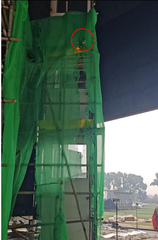
Photo 7-5 (a): Small Fires Spreading Along Safety Nets, Forming Flaming Droplets
