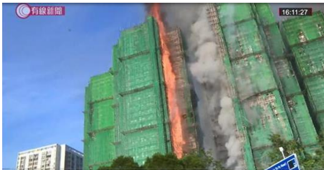
Photo 6-7 (e): Fire Spread Vertically throughout Wang Tao House
