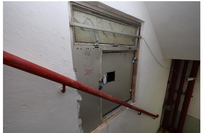
Wang Chi House Rear staircase between 19/F & 20/F
