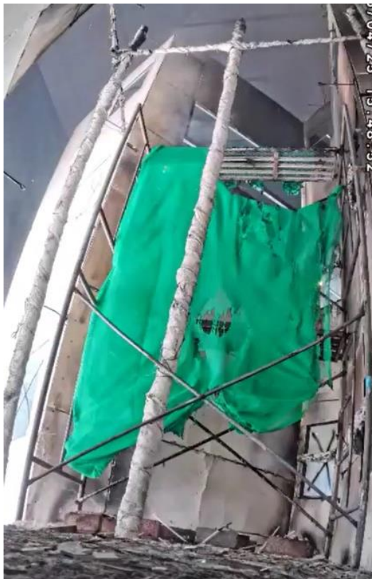
Photo 7-4 (d): Post-Fire Condition of Sample 2 (Partially Intact)
