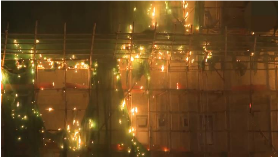
Photo 6-10: Flaming Droplets From Burning Safety Nets
