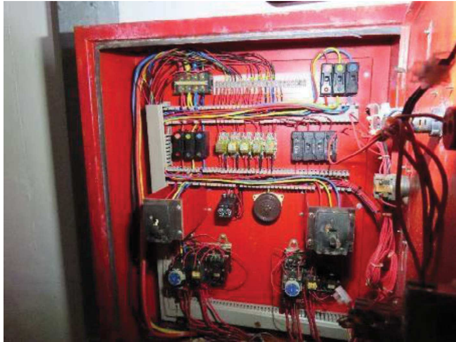
Photo showing the control panel wiring of fire booster pump control panel
