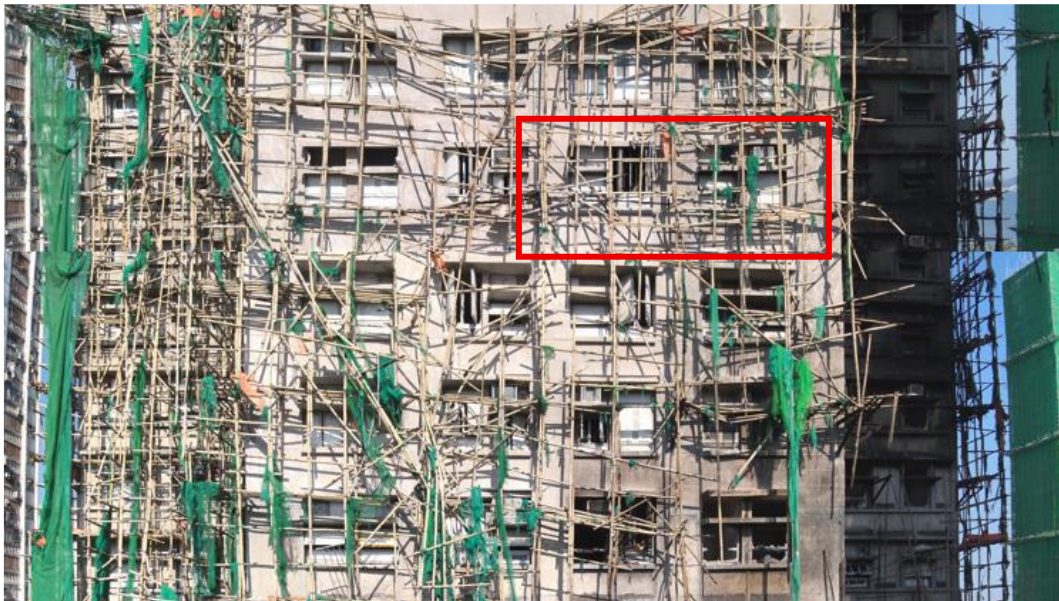
Photo 8-6 (f): External View of the Living Room Window of Flat 03
