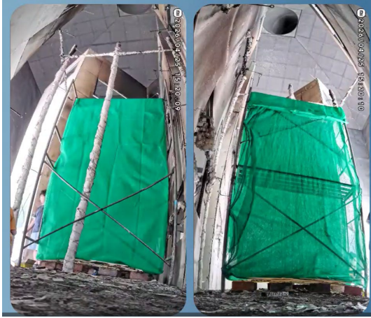
Photo 2-8: The Mobile Platform Setup (Fire Behaviour of Safety Nets)
