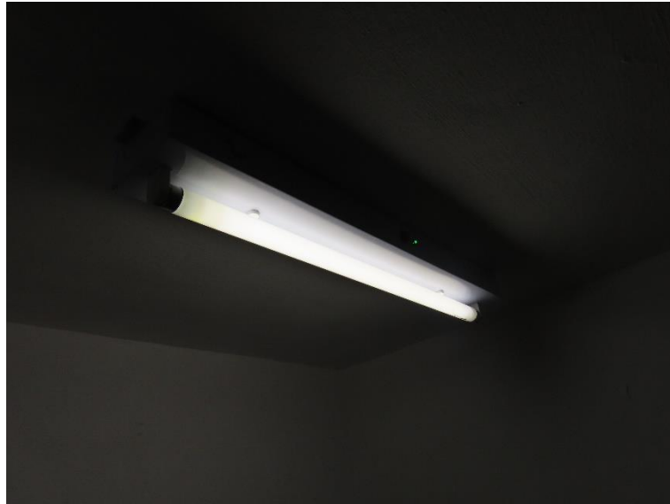
Photo showing the fluorescent tube-type emergency light Wang Chi House (Photo taken on 1.12.2025)
