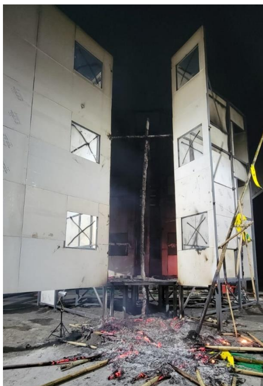
Photo 7-6 (g): Post-Fire Condition in Test 13 Using Safety Nets Collected From Wang Chi House and Non-FR Canvas
