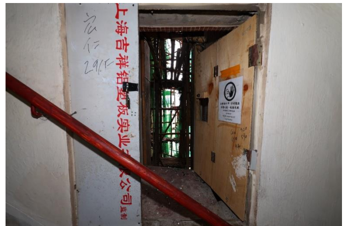
Wang Yan House Front staircase between 28/F & 29/F
