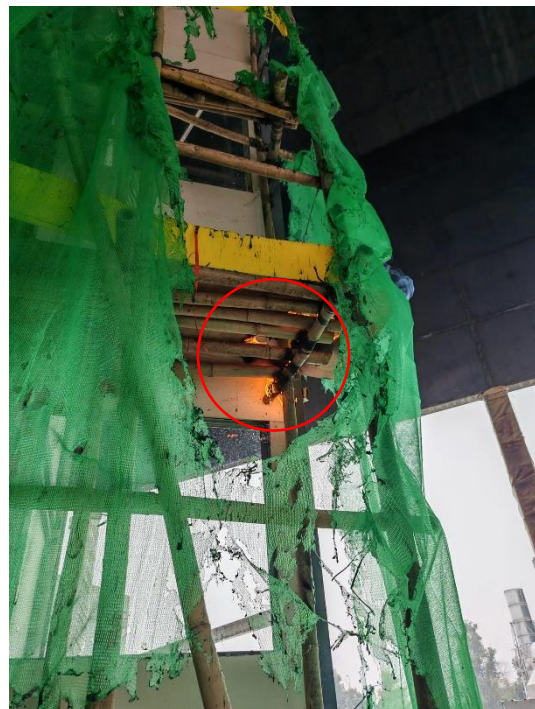
Photos 7-5 (g) & (h): Flaming Droplets Causing Further Fire Propagation
