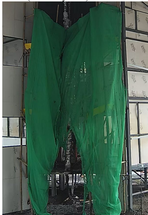
Photo 2-2 (d): No Secondary Ignition Occurred in Test 4
