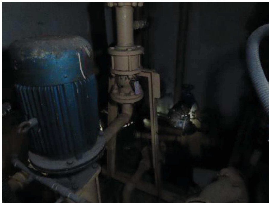
Photo showing the upfeed water pump
