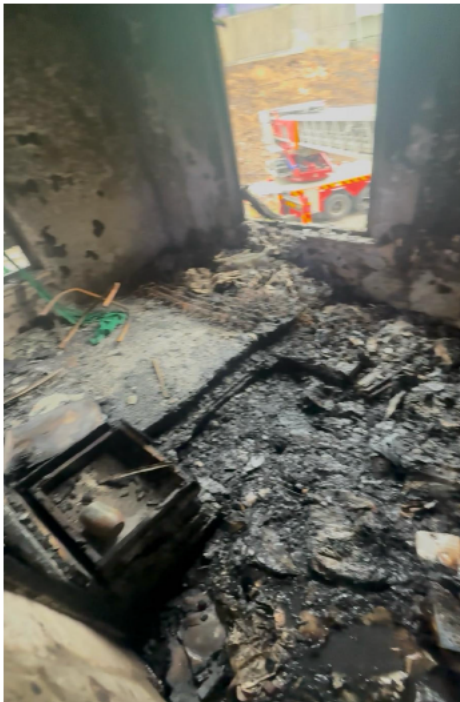
Bedroom 2 of Flat 104 Overview (Photo A11)
