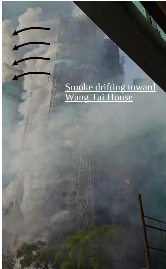
Photo 5-6 (f): Heavy Smoke on the South-East Façade at 1508 Hours
