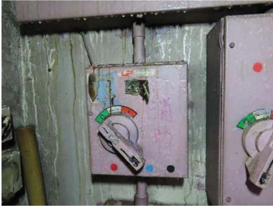
Photo showing the main switch of upfeed water pump (Power off position)
