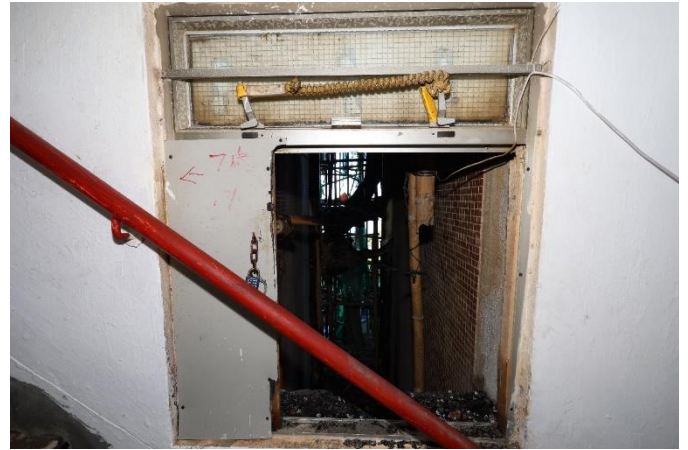
Wang Shing House Rear staircase between 9/F & 10/F
