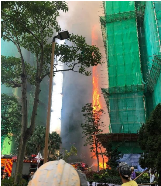
Photo 5-7 (a): Fire Spreading Along the West Re-Entrant at 1509 Hours
