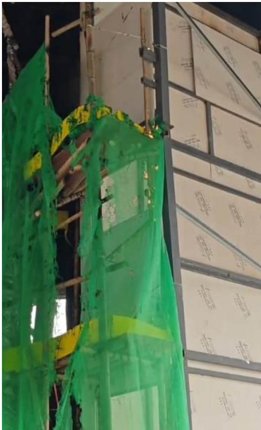
Photos 8-20 (c) & (d): Other Combustibles (Toe-Boards and Wooden Boards) Alight
