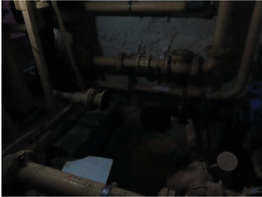
Photo showing the piping of upfeed water pump (Disconnected)
