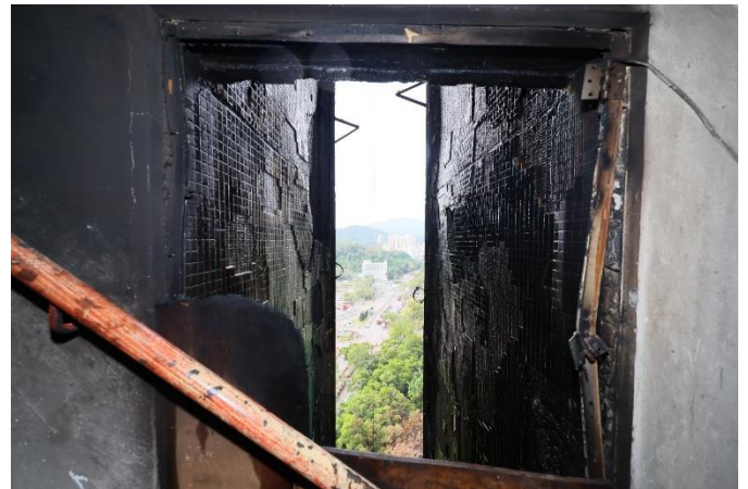
Wang Tai House Front staircase between 20/F & 21/F
