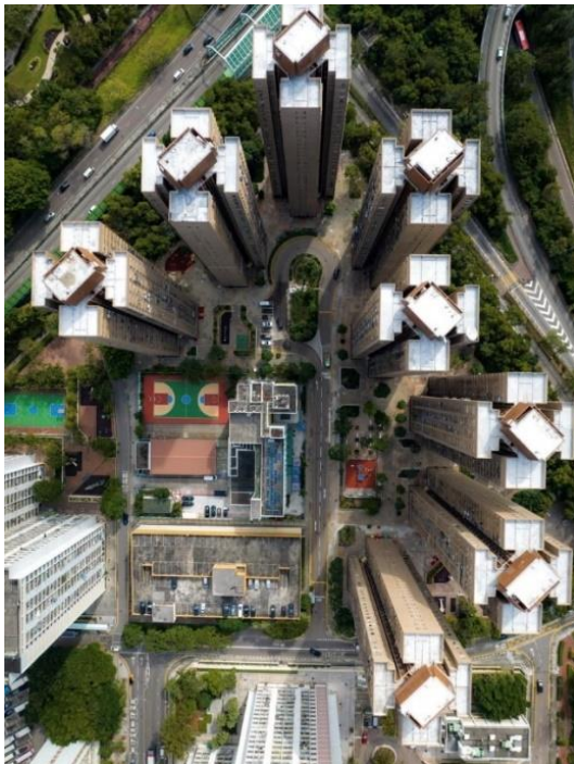
Photo 4-1 (a): Wang Fuk Court (Photo Taken in 2023) 7
