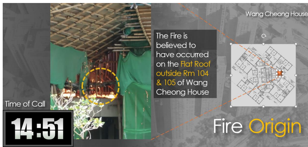
Figure A18-1 – Showing the Fire Origin at Flat Roof outside Flat 104 and 105 of Wang Cheong House
