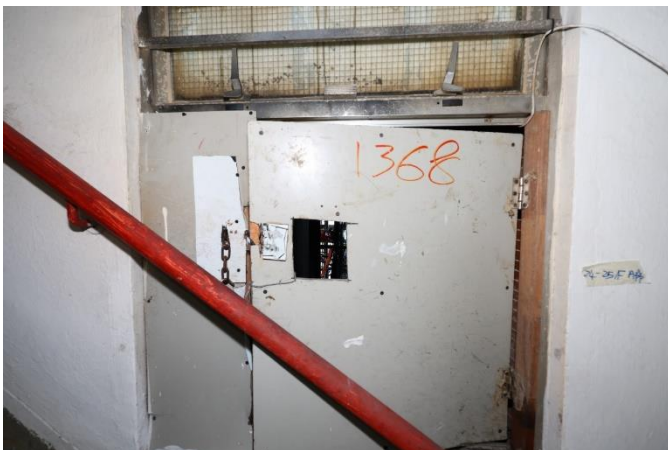
Wang Shing House Front staircase between 24/F & 25/F
