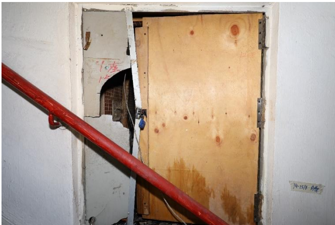
Wang Shing House Front staircase between 14/F & 15/F
