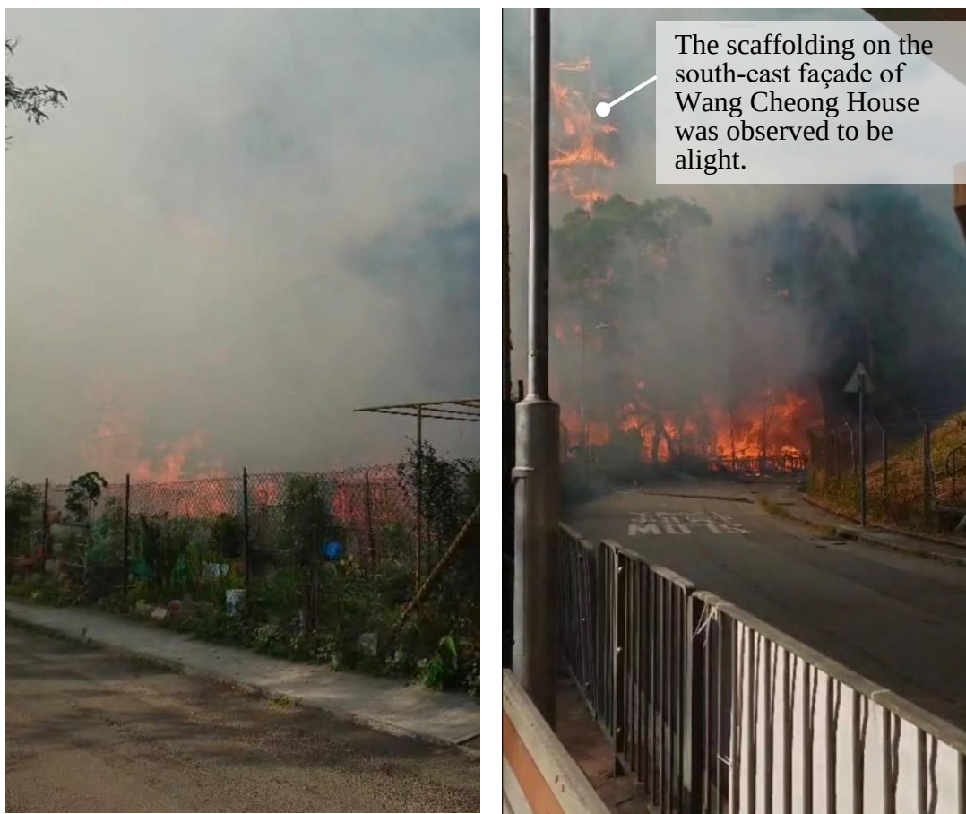
Photos 5-6 (a) & (b): Fire Spread to the Open Ground outside the South-East Façade of Wang Cheong House at About 1501 Hours
