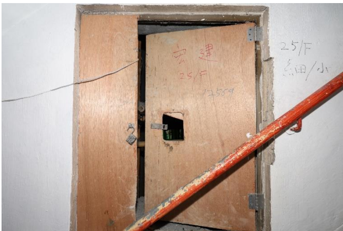
Wang Kin House Front staircase between 24/F & 25/F
