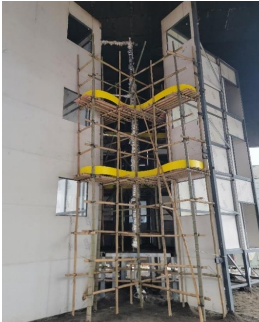
Photo 7-1 (b): Scaffolding Setup
