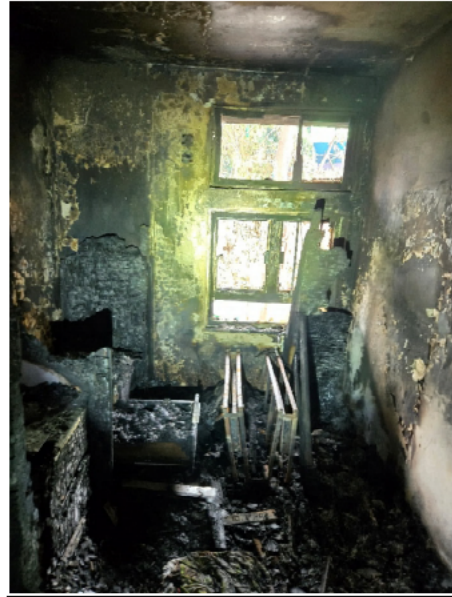
Bedroom 1 of Flat 104 Overview (Photo A10)
