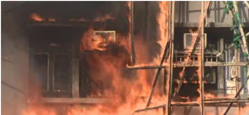
Photos 8-19 (d) to (f): Burning of Combustible Envelope Observed During the Fire
