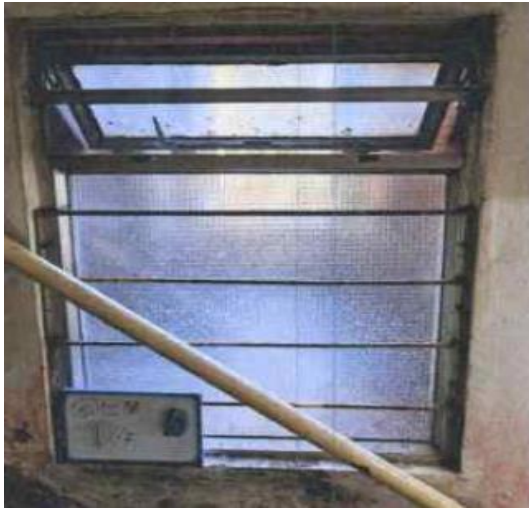
Photo 4-3 (a): Staircase Window (Before the Renovation Works)
