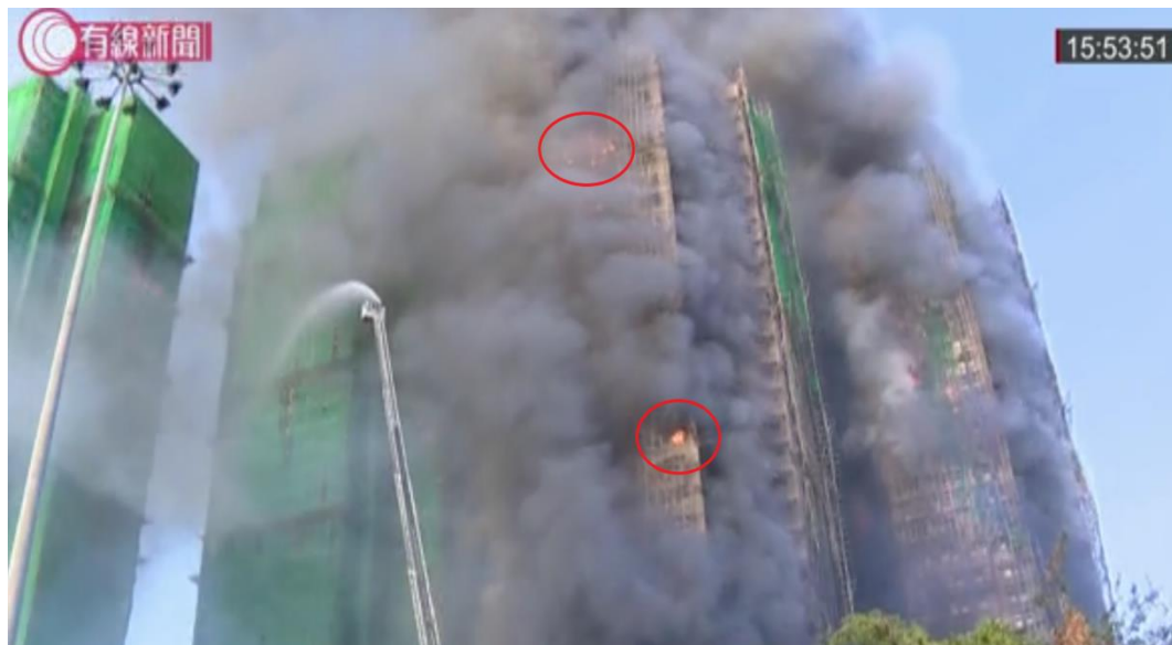
Photo 5-12: Flames From Ignited Units on the South-West Façade of Wang Tai House
