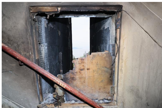
Wang Cheong House Front staircase between 10/F & 11/F
