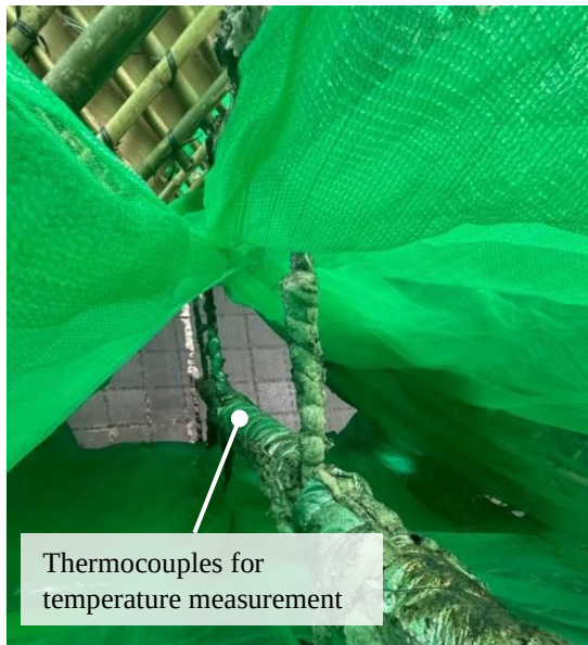
Photo 7-1 (e): Internal View With Safety Nets
