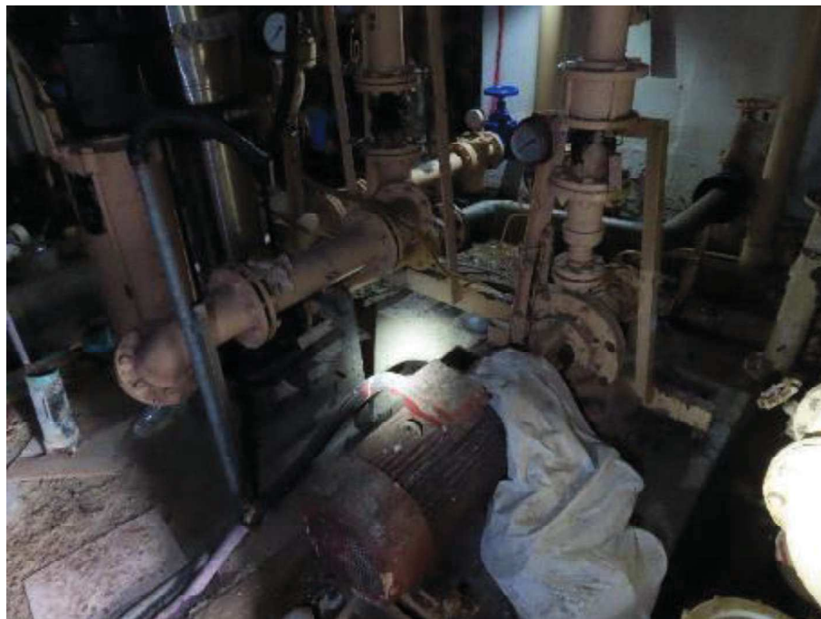
Photo showing the new installed upfeed water pump
