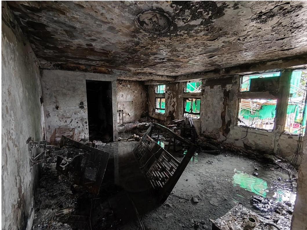
Photo 8-3 (a): Unit Sustained Extremely Severe Damage – Flat 02, Wang Yan House
