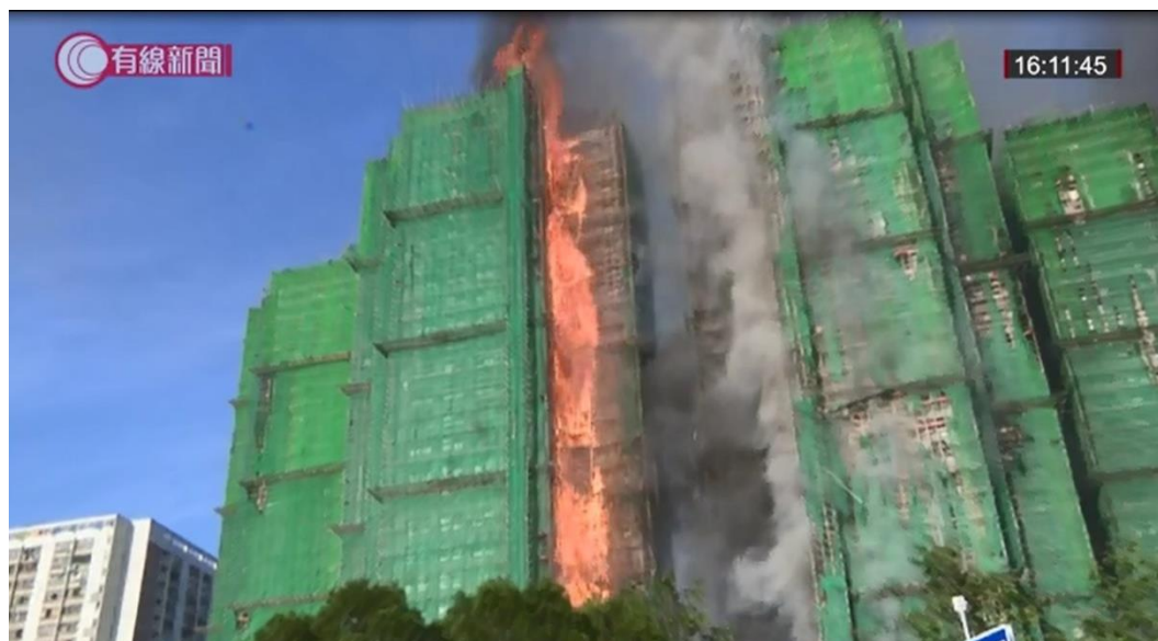
Photo 8-14: Flames From the Re-Entrant Observed Rising Higher Than the Building at Wang Tao House
