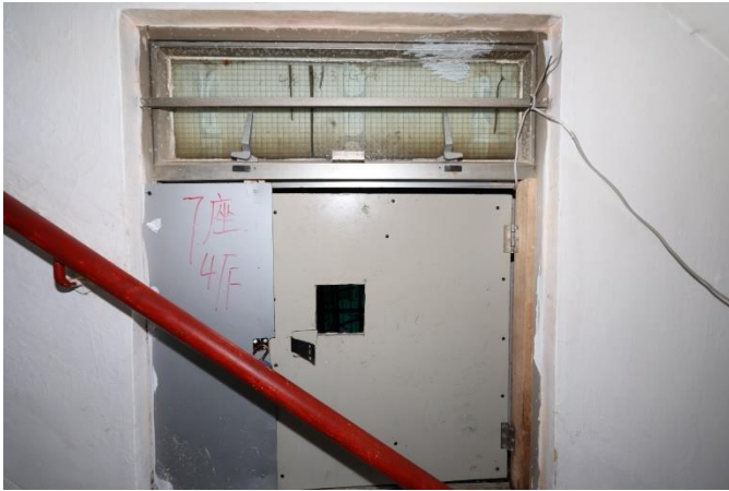
Wang Shing House Rear staircase between 3/F & 4/F
