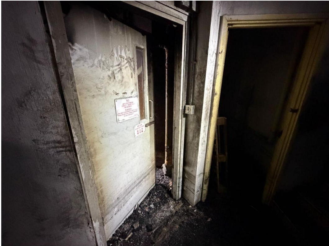
Photo 4-1 (b): Rear Exit at Wang Cheong House
