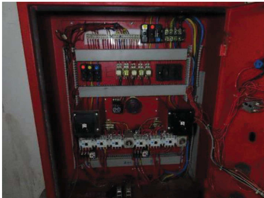
Photo showing the control panel of fire booster pump (Power unavailable)
