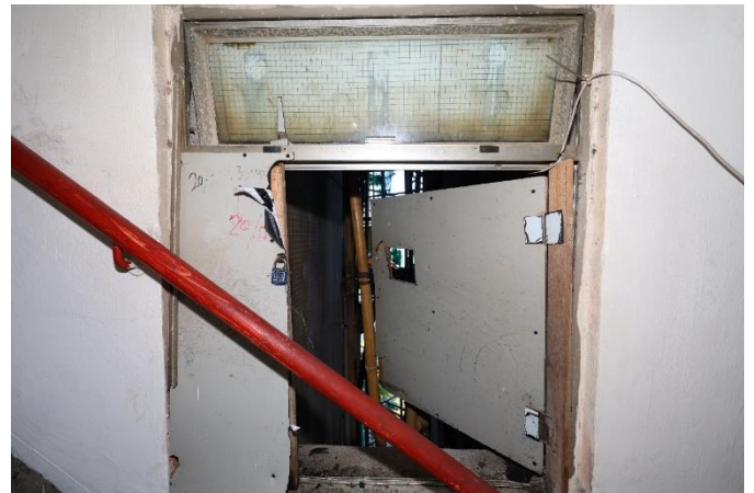
Wang Shing House Rear staircase between 19/F & 20/F
