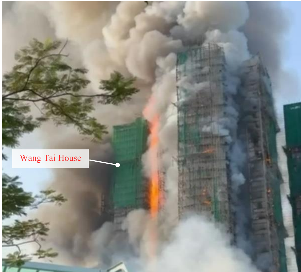
Photo 9-4: Rapid Vertical Fire Spread Along the East Re-Entrant of Wang Tai House at 1516 Hours
