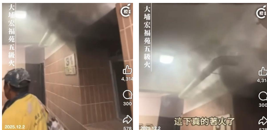
Photos 10-7 (a) & (b): Video From Online Source Showing Smoke Entering Lift Lobby Through the Upper Openable Part of Window of Wang Tai House
