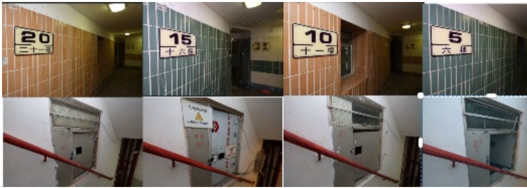
Photo: Other situations on fifth, tenth, fifteenth, and twentieth floors of Wang Chi House
