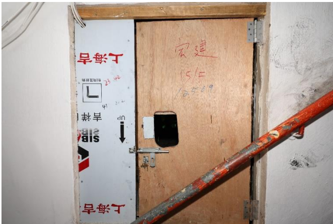
Wang Kin House Rear staircase between 15/F & 16/F
