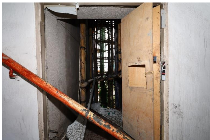
Wang Tao House Rear staircase between 15/F & 16/F
