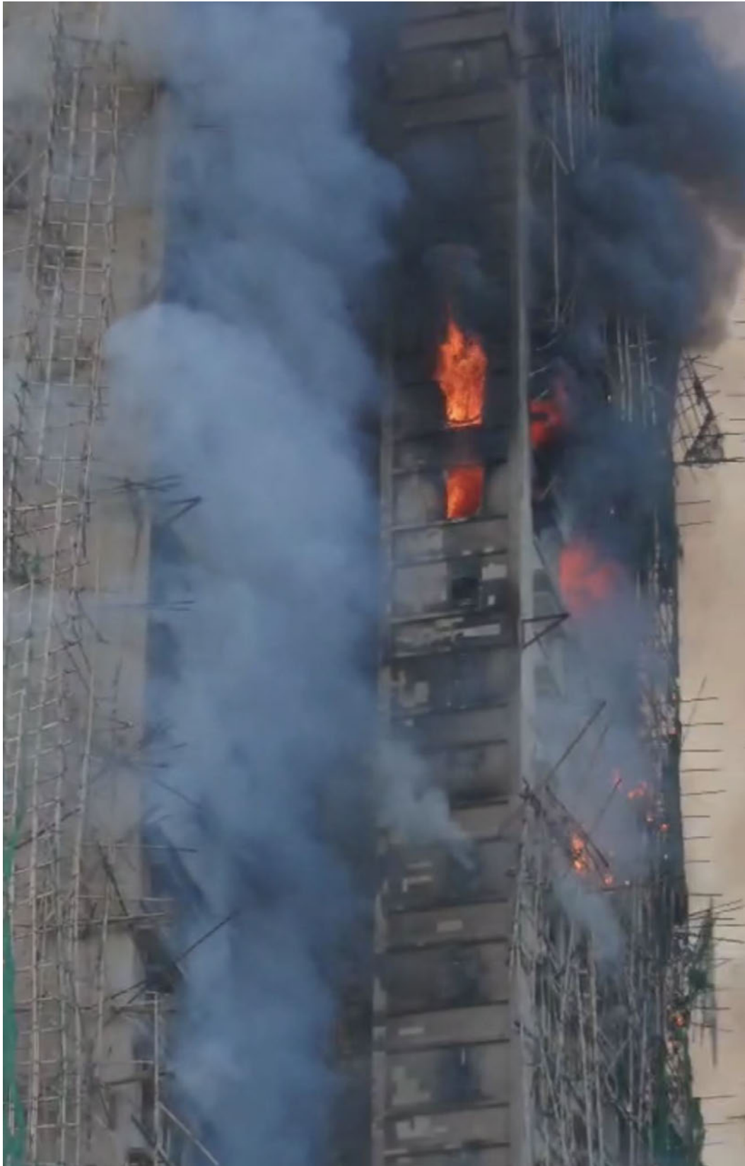
Photo 10-3 (c): The Bamboo of the Scaffolding on Southeast Façade of Wang Cheong House Fell and Possibly Blocked the Rear Exit
