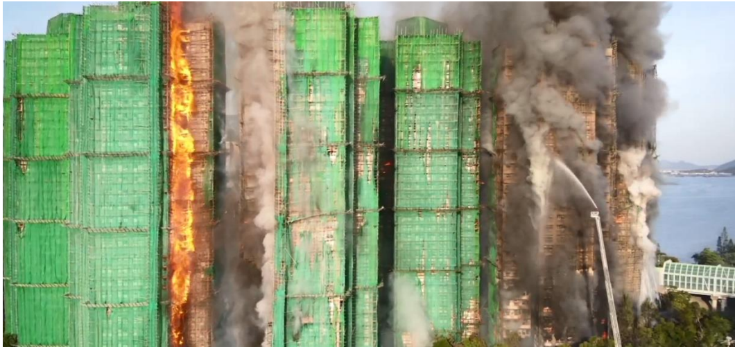
Photo 10-1 (a): Rapid Vertical Fire Spread Along Re-Entrant of Wang Tao House
