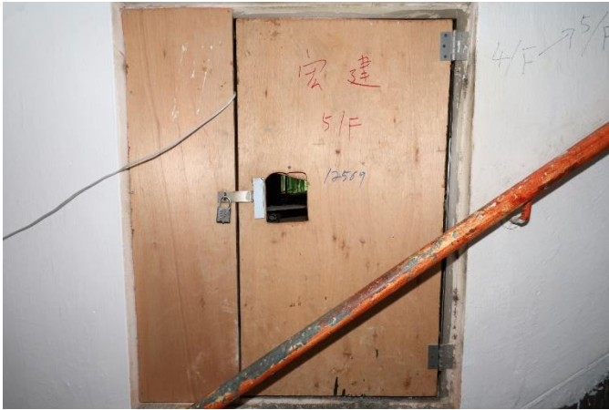
Wang Kin House Front staircase between 4/F & 5/F
