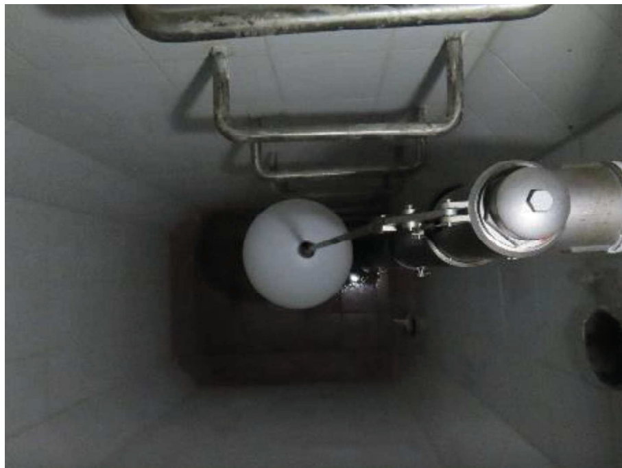
Photo showing the F.S. Up-feed tank of upfeed water pump (Water unavailable)
