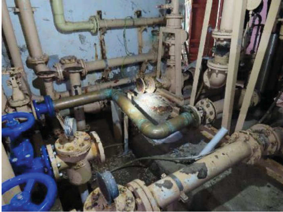
Photo showing the new installed piping of upfeed water pump
