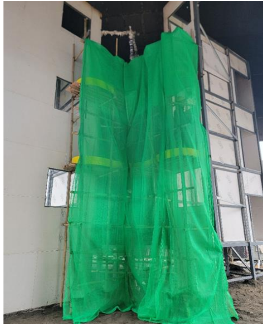
Photo 7-1 (c): External View With Safety Nets
