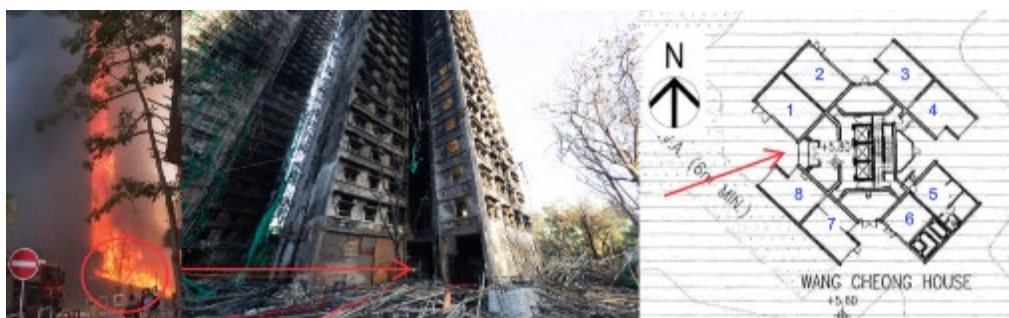
Photo: Ground floor fire plume 2 at building entrance and resulting damage following the incident at Wang Cheong House
