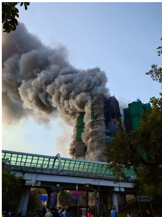
Figure 5 (c): Heavy Smoke on the South Re-entrant of Wang Cheong House at 1537 hours
