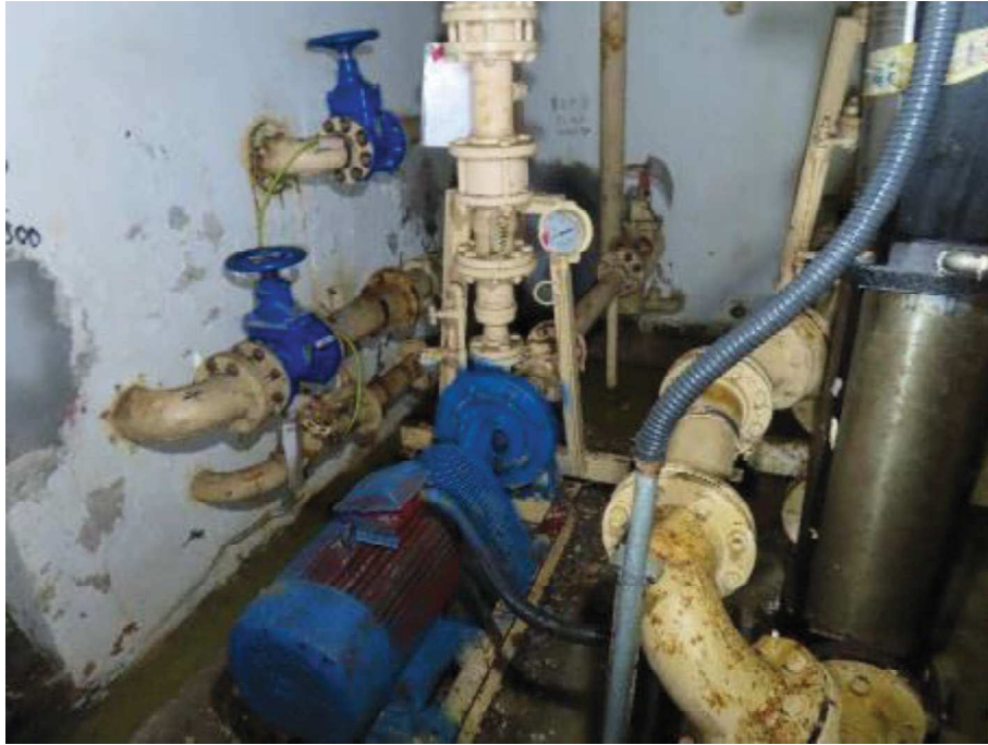
Photo showing the upfeed water pump and piping
