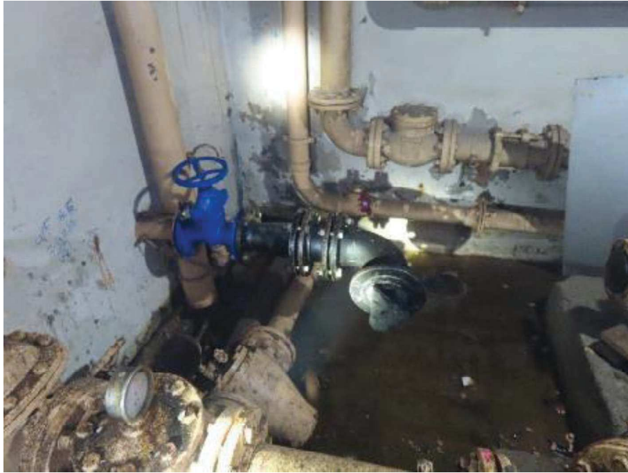
Photo showing the new installed piping of upfeed water pump (Disconnected)
