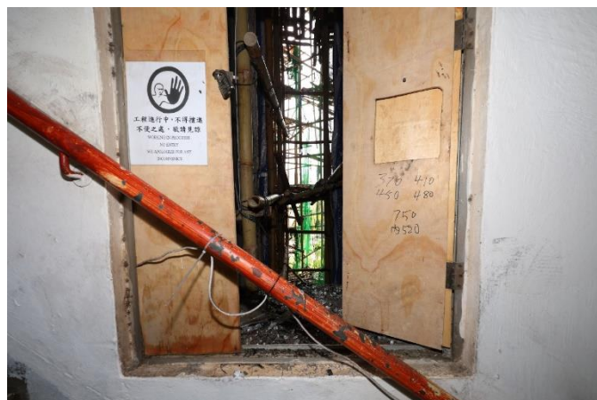
Wang Tao House Front staircase between 10/F & 11/F
