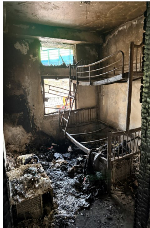
Bedroom 2 of Flat 105 Overview (Photo B12)
