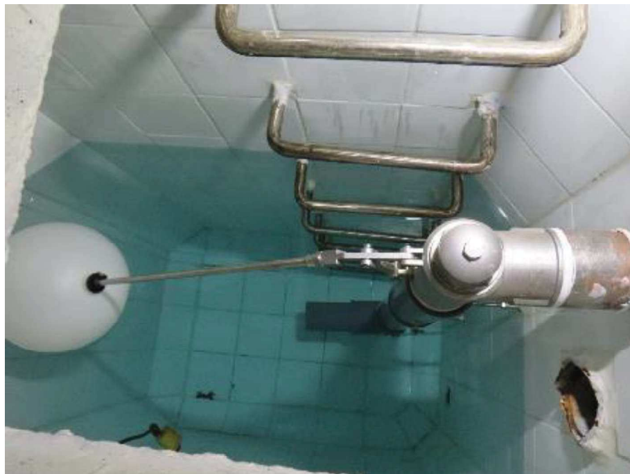
Photo showing the F.S. Up-feed tank of upfeed water pump (Water available)
