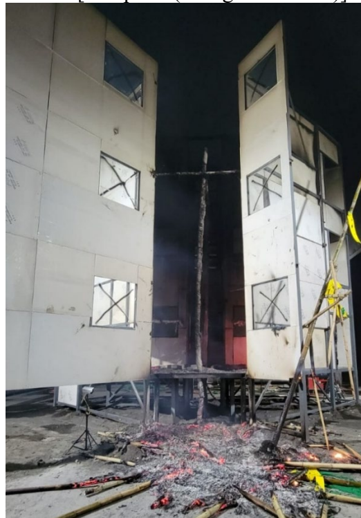
Photo 2-16 (p): Post-Fire Condition in Test 13 [Sample 4 (Wang Chi House)]
