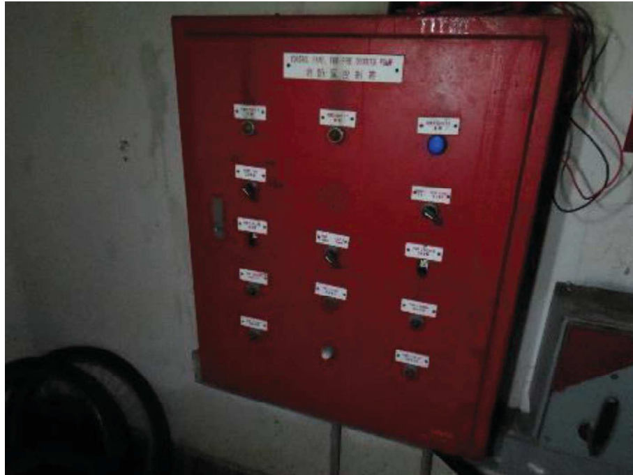
Photo showing the control panel of fire booster pump (Power unavailable)
