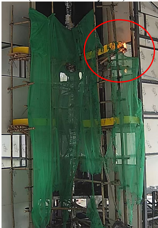
Photo 2-2 (c): Secondary Ignition Occurred in Test 3
