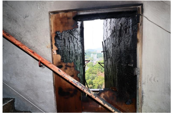
Wang Tai House Front staircase between 10/F & 11/F
