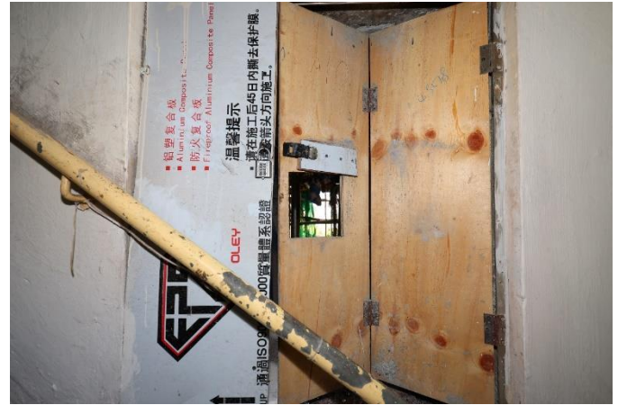
Wang Yan House Front staircase between 8/F & 9/F
