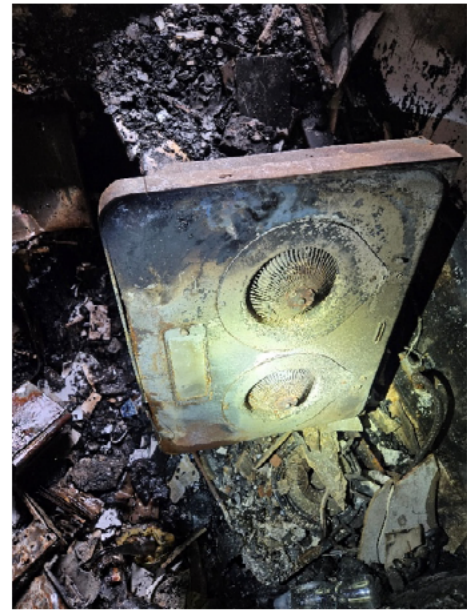
Range Hood in Kitchen of Flat 104 (Photo A8)
