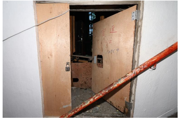
Wang Kin House Rear staircase between 9/F & 10/F
