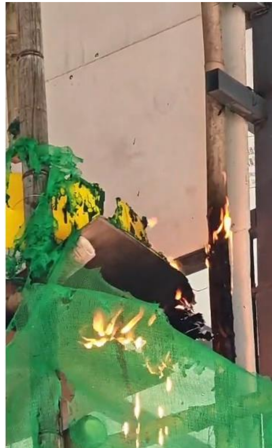
Photos 8-20 (c) & (d): Other Combustibles (Toe-Boards and Wooden Boards) Alight
