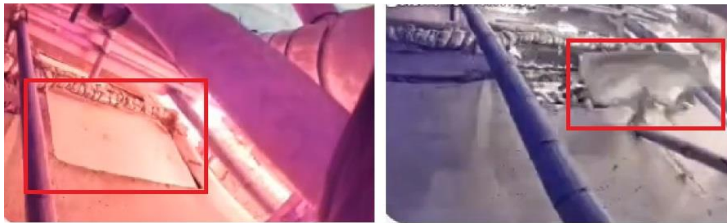
Photo 10-6 (b): Polystyrene Panel Detached From Building Exterior
